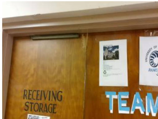
Interior Wood Door
