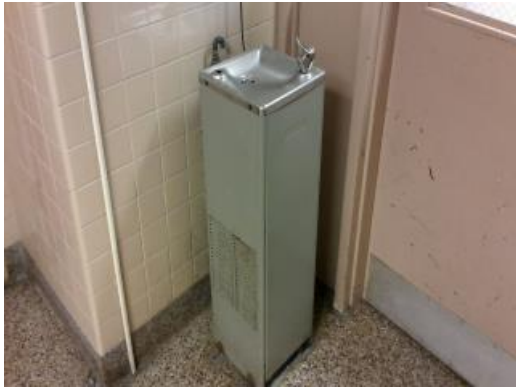
Original Water Cooler
