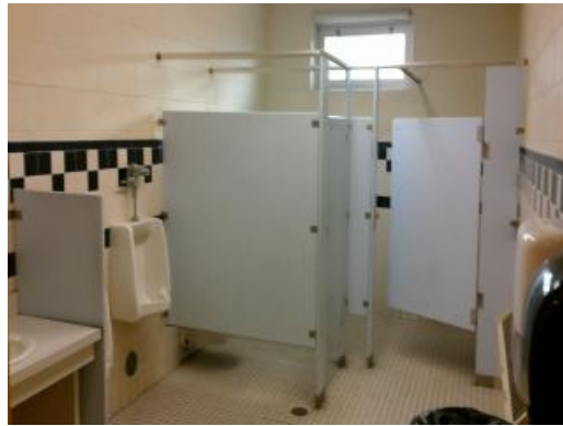
Restroom Fixtures And Finishes
