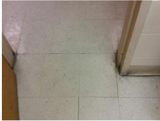
Separating VCT Flooring
