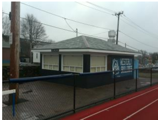
Building 04 - Concession Stand
