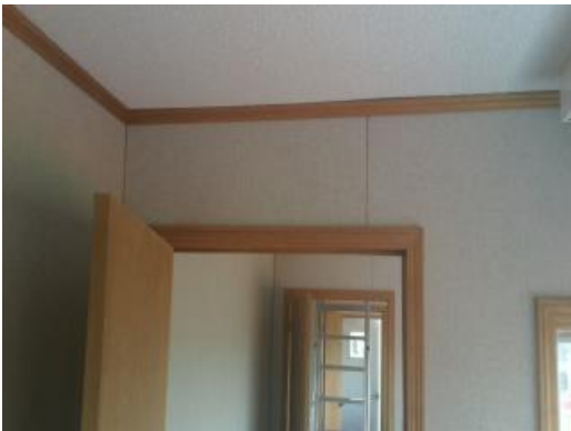
Building 03 - Gypsum Ceiling
