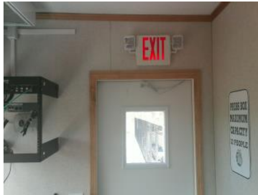
Building 03 - Exterior Steel Door
