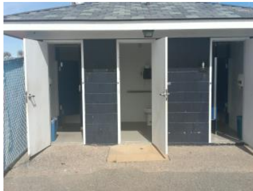
Building 04 - Back Bathroom Area
