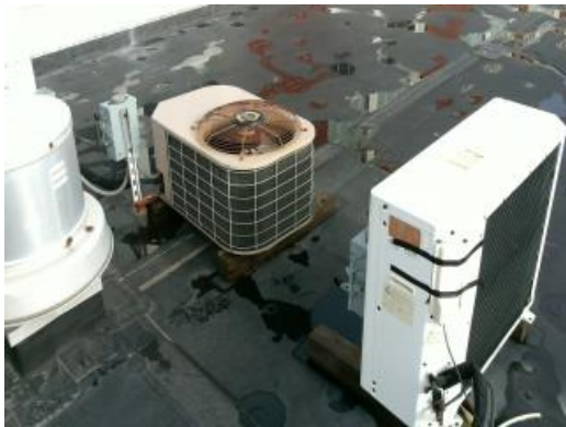
Main Building - Abandoned Equipment
