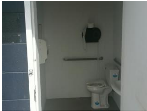
Building 04 - Back Bathroom ADA
