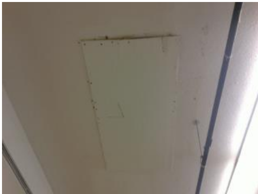
Main Building - Cafeteria Ceiling
