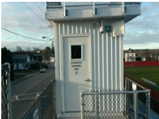
Building 03 - Exterior Door
