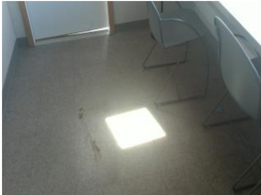
Building 03 - VCT Flooring
