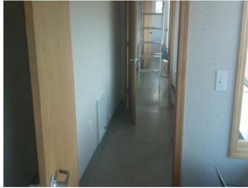
Building 03 - Interior Wood Doors
