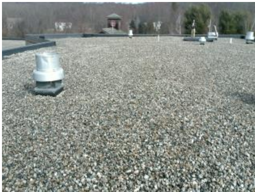
Ballasted Roof
