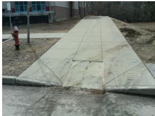
Concrete Pedestrian Paving
