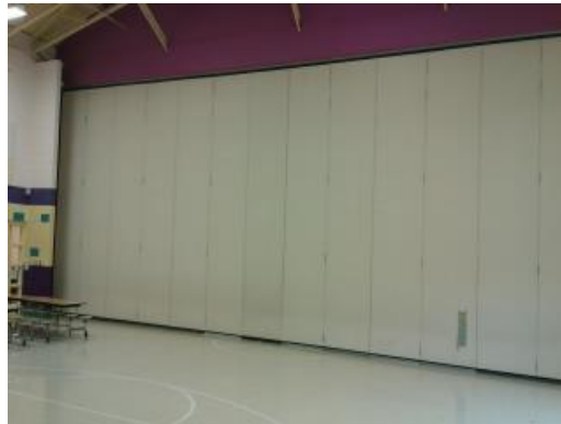
Gymnasium Partition Wall
