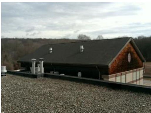
Steep Slope Roof
