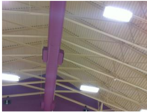
Exposed Gym Ceiling
