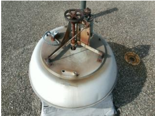
Large Exhaust Fan Missing Cover
