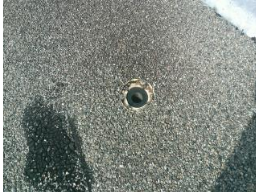
Missing Drain Cover
