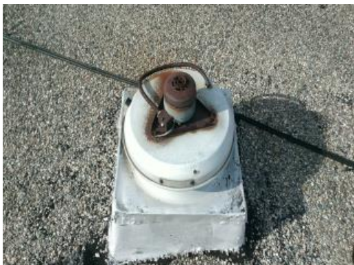
Damaged Small Exhaust Fan
