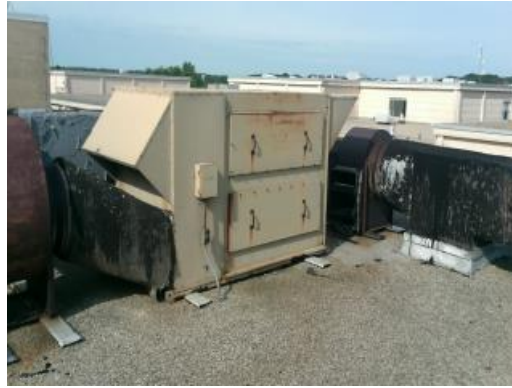
Weathered Package Unit
