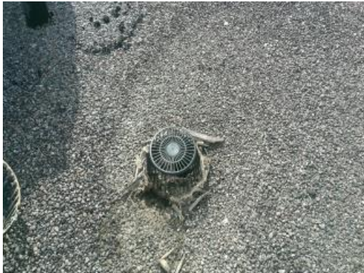
Debris In Roof Drain
