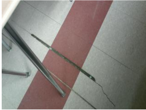
Cracked Flooring
