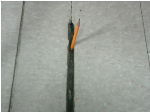
Crack In VCT Floor
