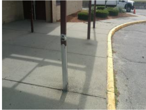
Damaged Canopy Columns
