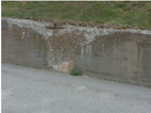
Deteriorated Concrete Retaining Wall
