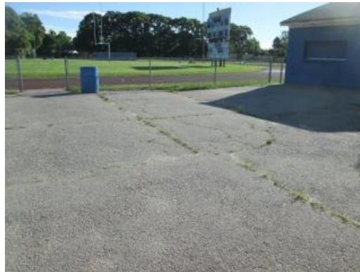
Asphalt Pedestrian Pavement
