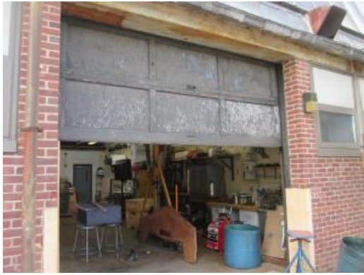
Shop Classroom Overhead Door
