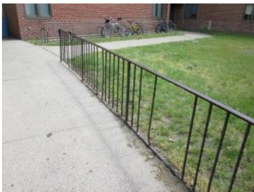
Main Entry Ornamental Fence
