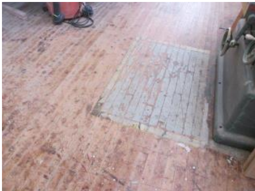
Shop Classroom Wood Floor
