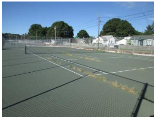
Tennis Court Paving
