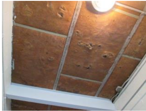
Exposed Insulated Panel Ceiling
