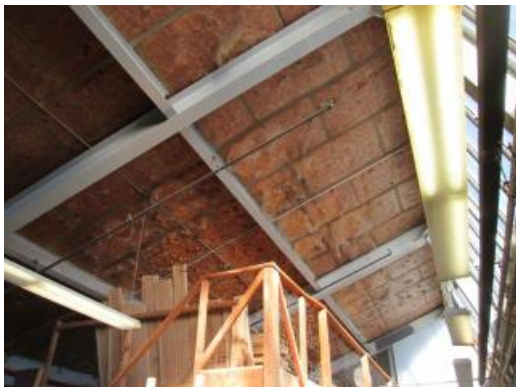
Exposed Insulated Panel Ceiling
