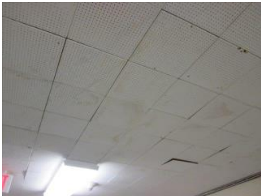
Adhered Ceiling Tiles
