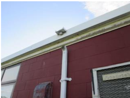
Damaged Downspout
