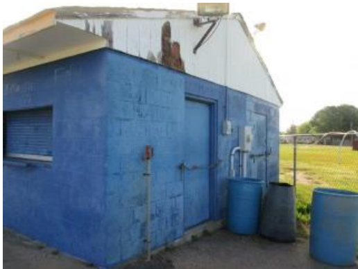
Back Side Exterior
