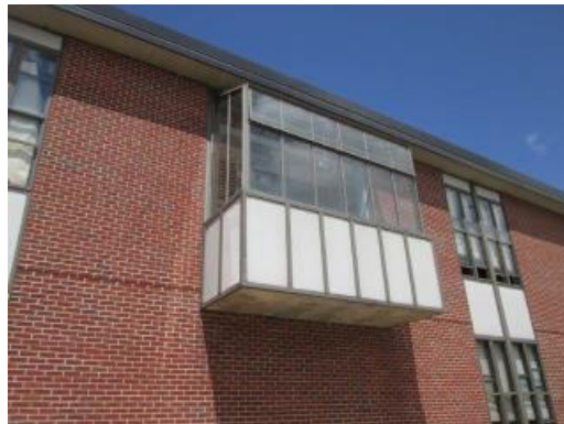
Bay Window At Science Prep Room
