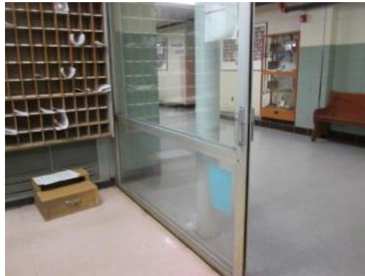
Main Office Sliding Glazed Doors
