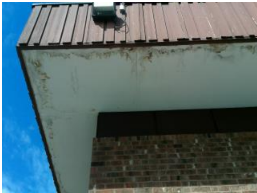
Damaged Soffit
