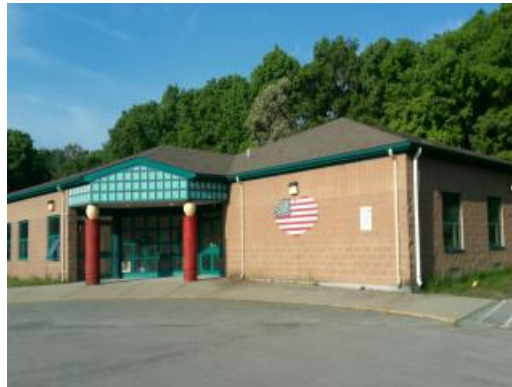
North Addition Exterior
