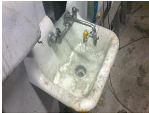
Stained And Corroded Service Sink
