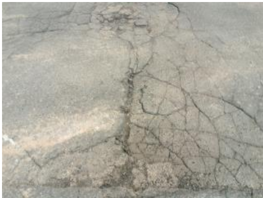
Cracked Roadway Asphalt
