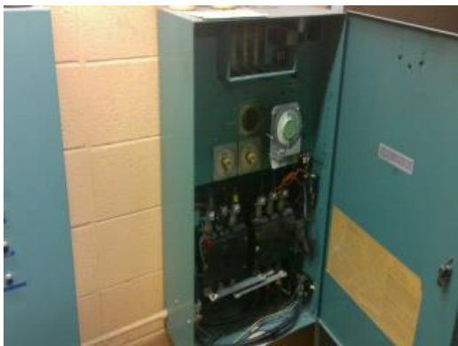
Transfer Switch With Burned Contacts
