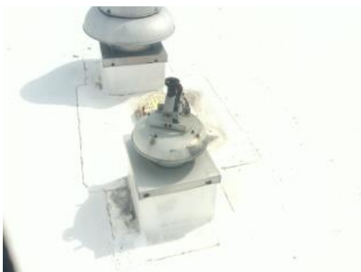
Damaged Small Exhaust Fan
