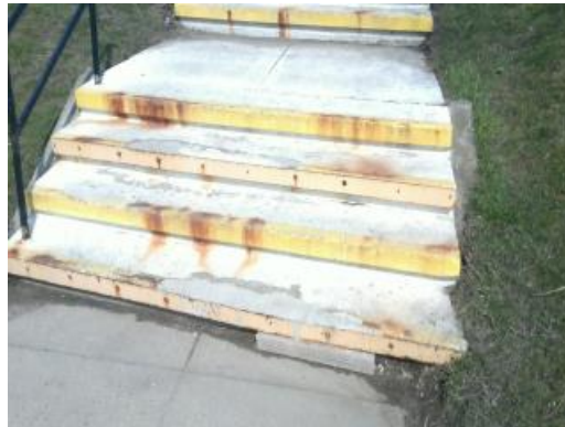
Concrete Stairs Settling
