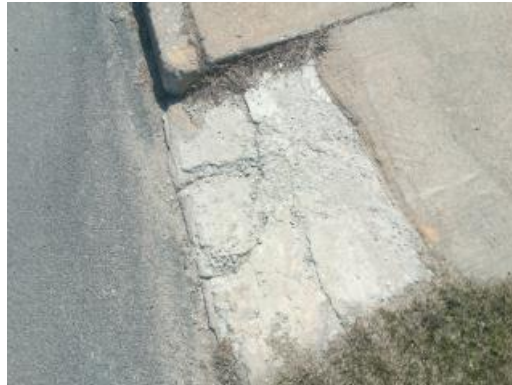
Cracked Concrete Walkway
