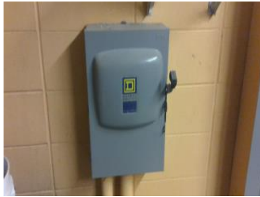
Transformer Disconnect
