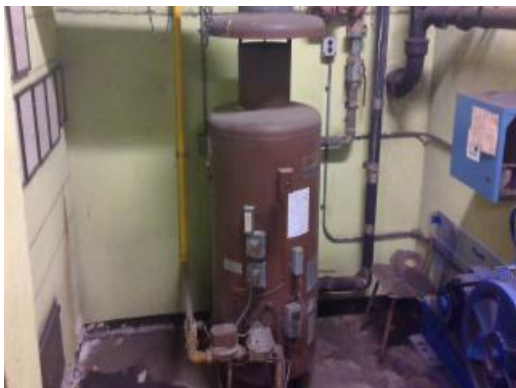
Aged Boiler For Hot Water
