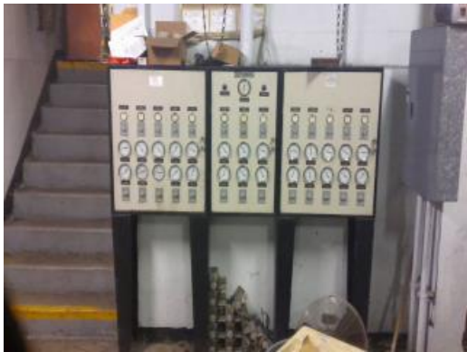
Pneumatic Controls Panel
