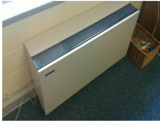
Non-Functional Heating Unit
