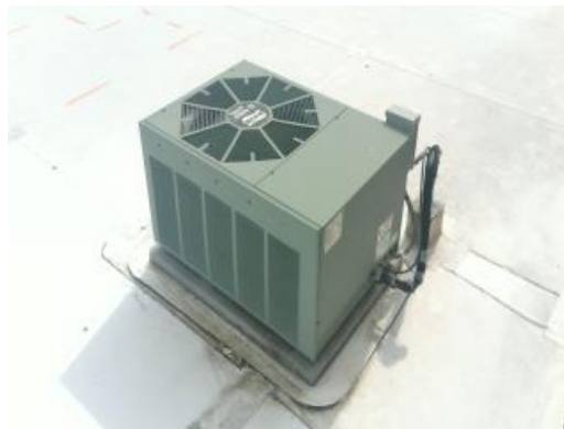
Condenser With Collapsed Coils
