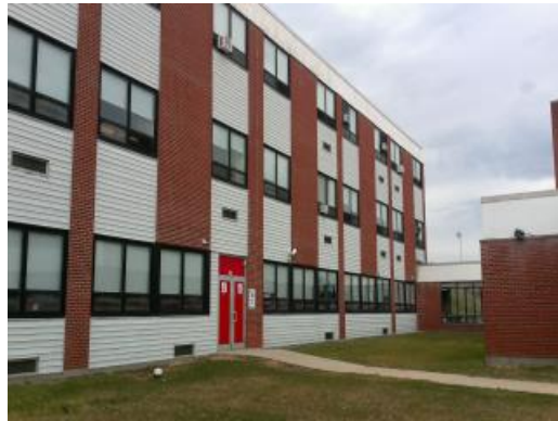
Typical Window Condition
