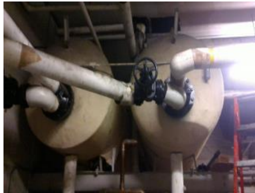
Original Water Storage Tank
