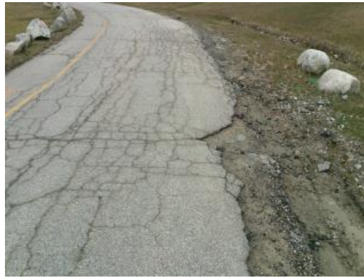
East Roadway Asphalt Paving
