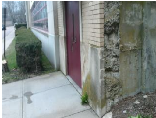
Concrete Wall Corner
