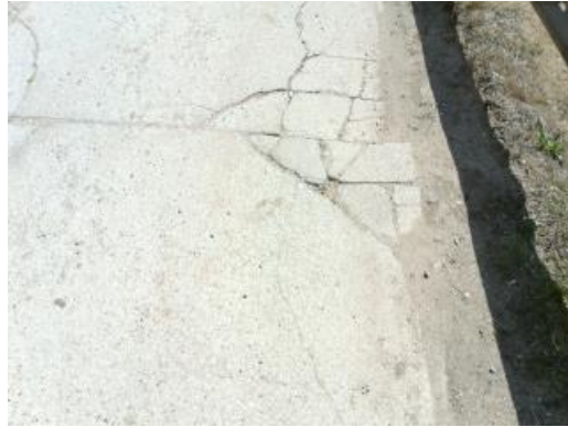
Cracked Sidewalks
