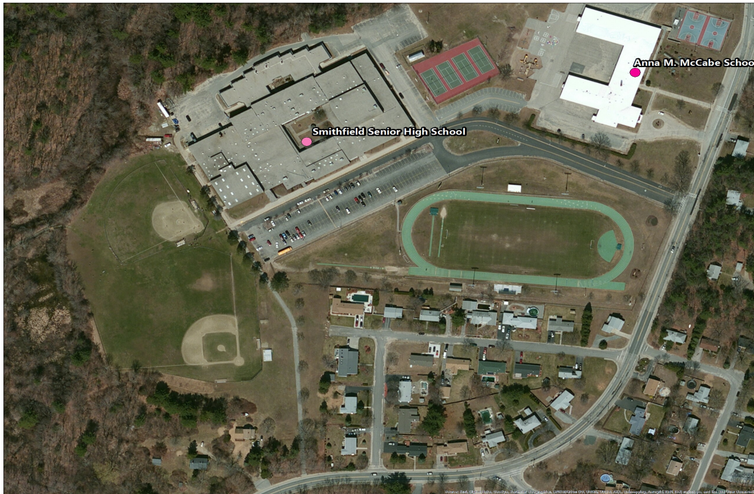
Figure 1: Aerial view of Smithfield Senior High School
