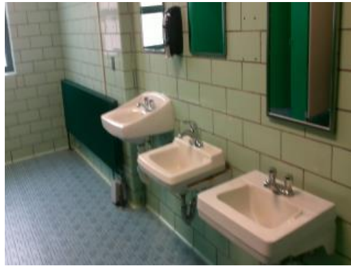
Typical Restroom Lavatories
