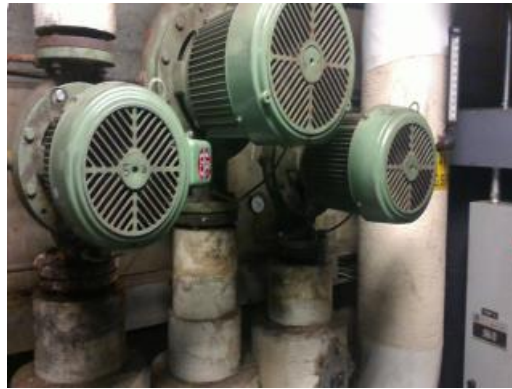
Corroded Pumps
