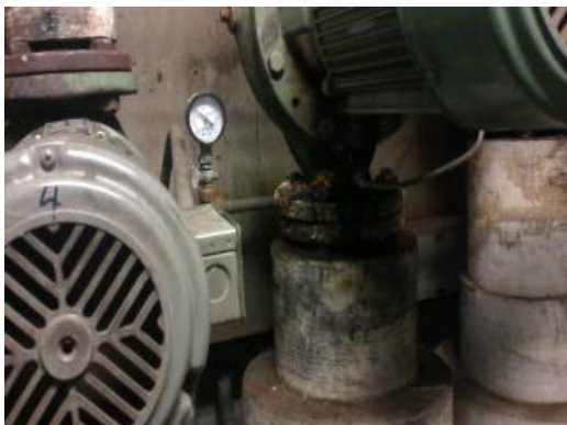
Corroded Pumps
