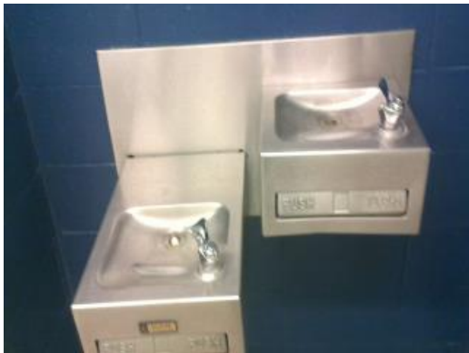
Damaged Drinking Fountains
