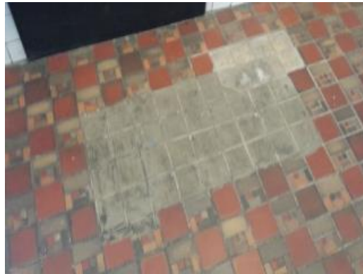
Worn And Missing Tiles
