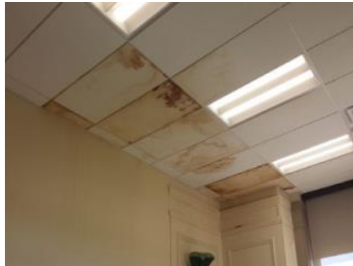
Stained Ceiling Grid And Tiles
