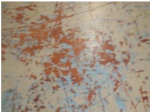
Peeling Concrete Floor Finish
