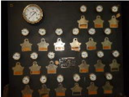
Pneumatic Control Panel
