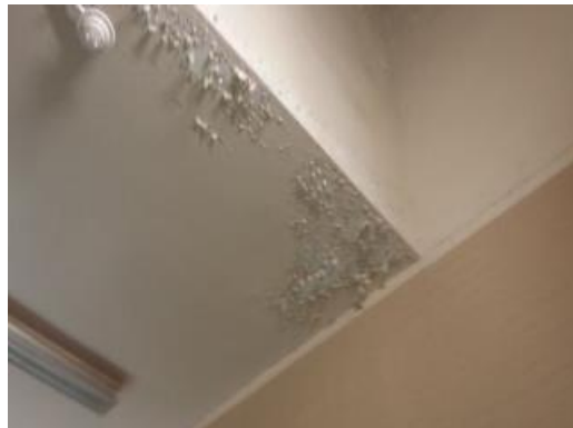
Peeling Ceiling Paint
