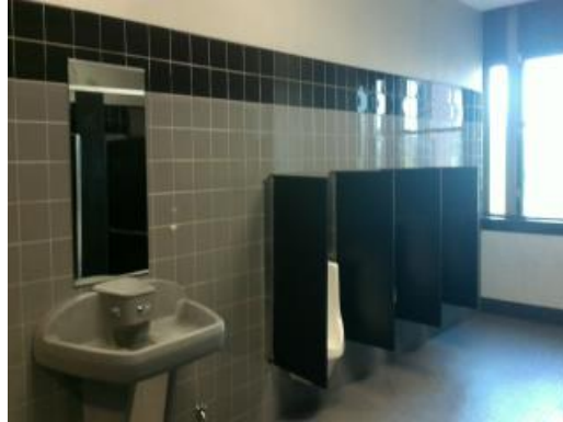
Restroom Fixtures And Finishes
