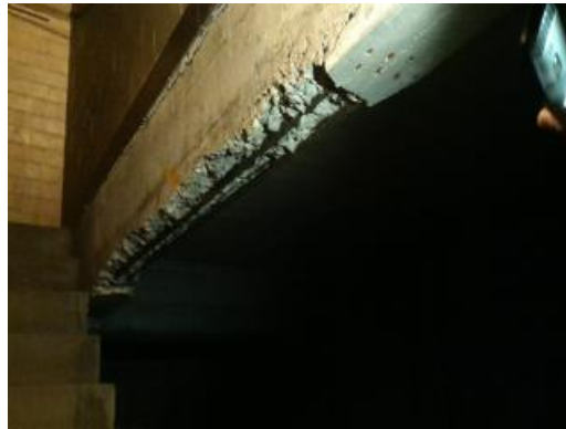
Concrete Beam Under Locker Rooms
