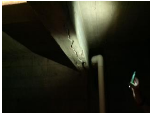
Concrete Beam Under Locker Rooms
