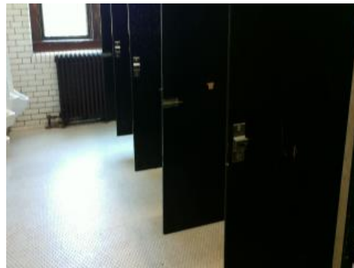
Typical Student Restroom
