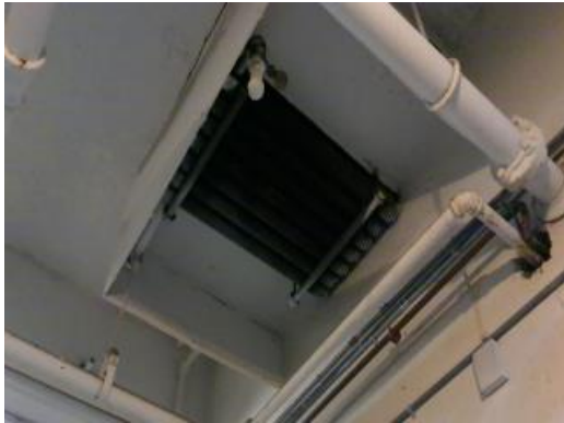
Ceiling Mounted Steam Coil
