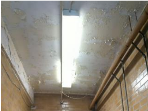
Basement Ceiling Damage
