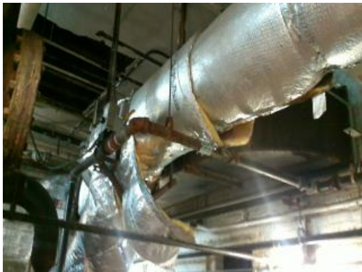
Damaged Insulation
