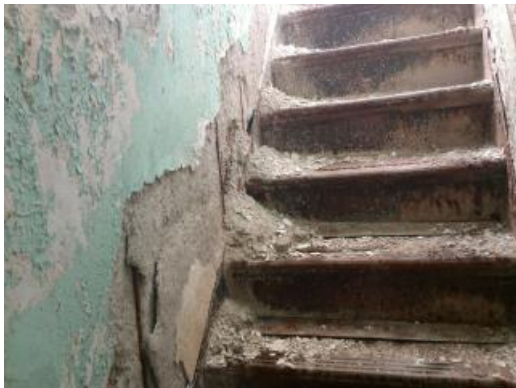
Bell Tower Stair
