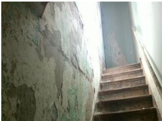
Bell Tower Stair
