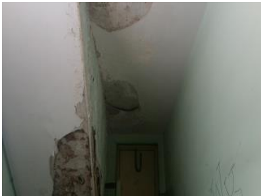
Bell Tower Stair
