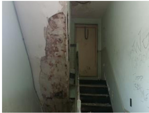
Bell Tower Stair
