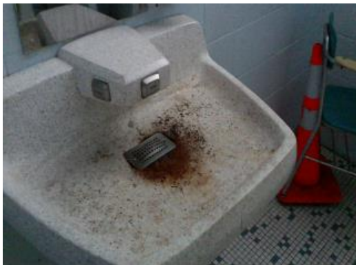
Rusted Bradley Half Sink
