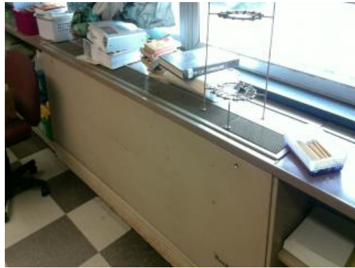
Typical Unit Vent Heat
