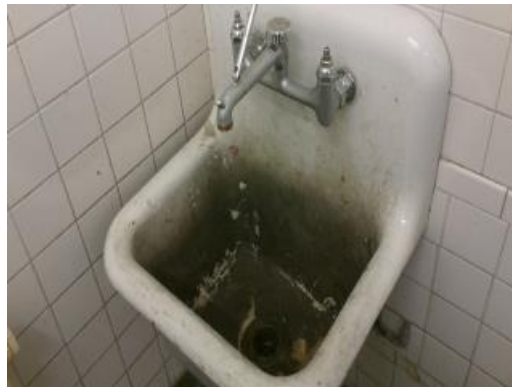
Typical Mop Sink
