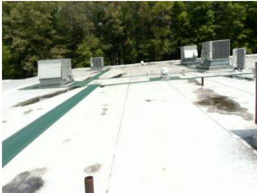
Typical Roof Condition
