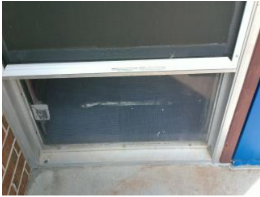
Original Single Pane Windows
