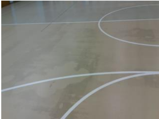
Gymnasium Sport Flooring
