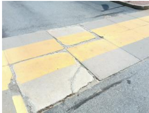
Concrete Walkway At Entrance
