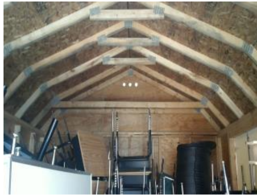
Storage Shed Interior
