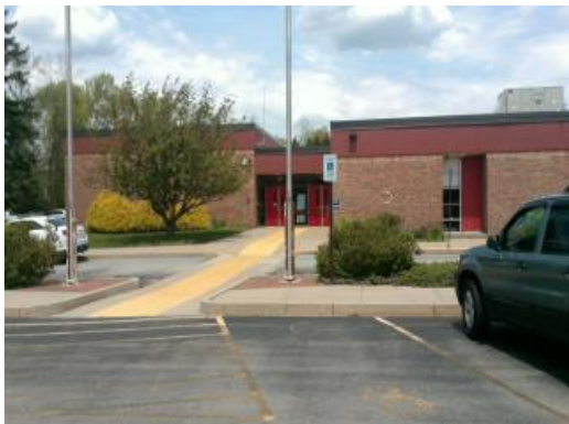
Front Of Building
