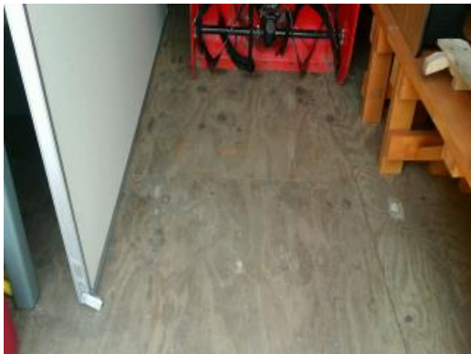
Storage Shed Floor
