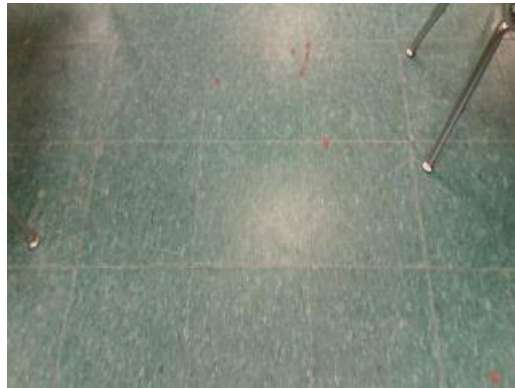
Faded And Worn VCT
