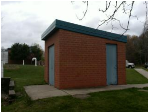
Utility Building Exterior
