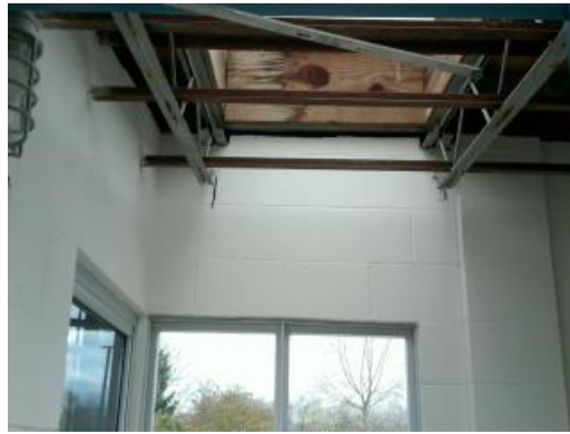
Ticket Booth Exposed Deck Ceiling
