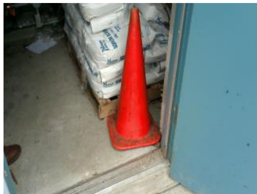
Utility Building Concrete Flooring
