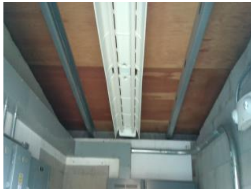
Utility Building-2 Wood Deck Ceiling
