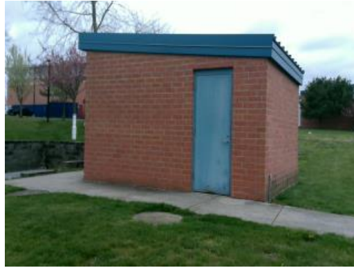
Utility Building Side
