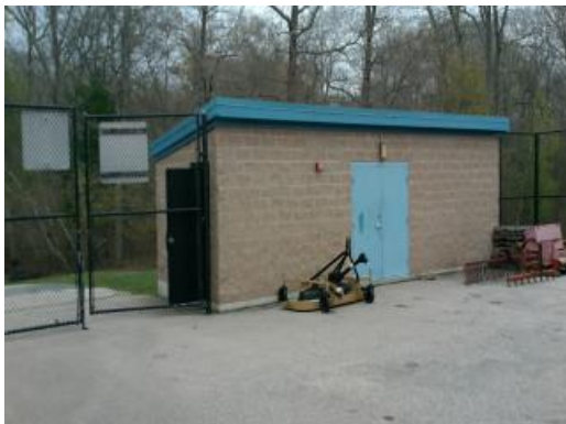
Storage Building Exterior
