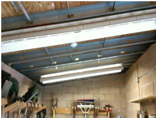
Storage Building Open Deck Ceiling
