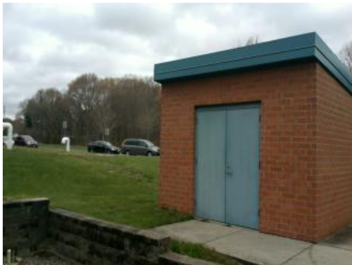
Utility Building Front
