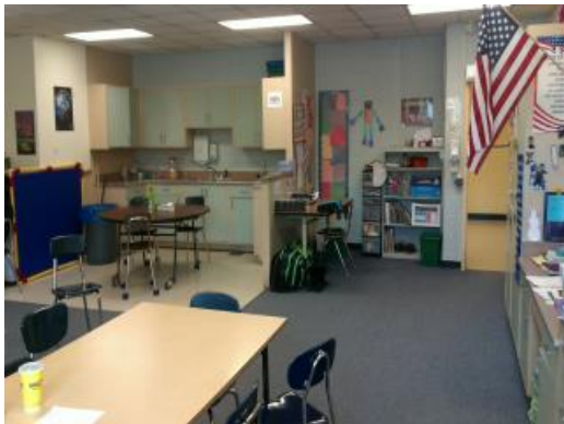
Worn Carpet at Classrooms
