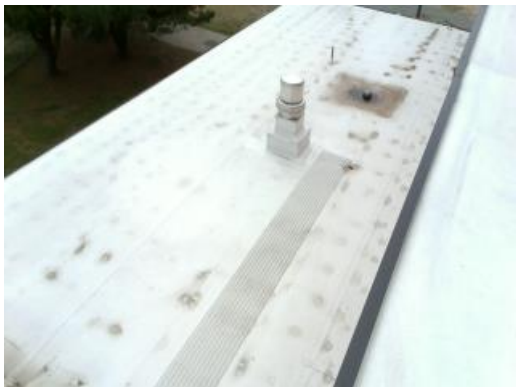
Roof Facing Faculty Parking
