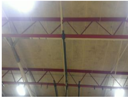
Stained Tectum Ceiling in Gymnasium
