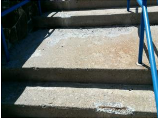
Steps Near Main Entrance
