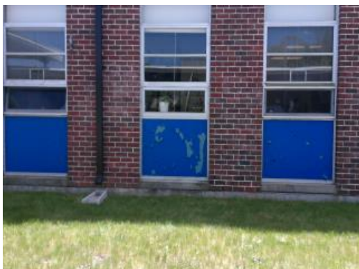
Typical Exterior Windows
