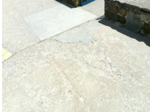
Spalling Sidewalk
