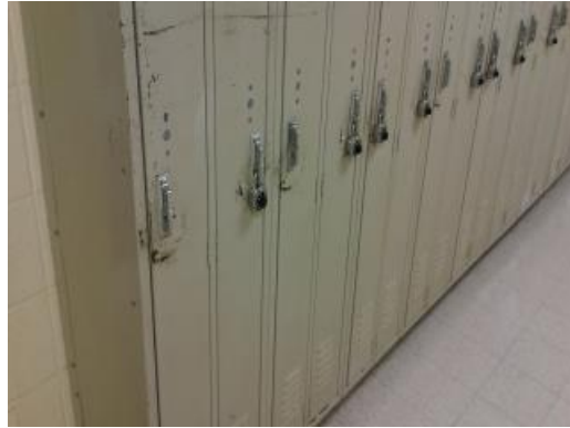
Corroded Lockers at Basement
