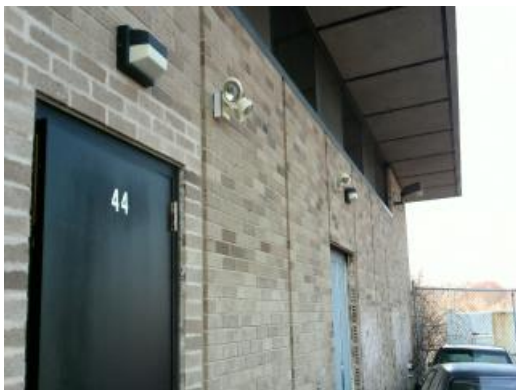
Building Mounted Lighting
