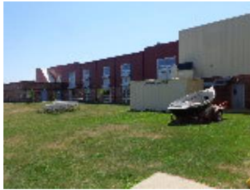
High School Wing Exterior
