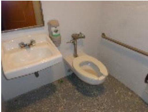
Restroom Fixtures And Finishes
