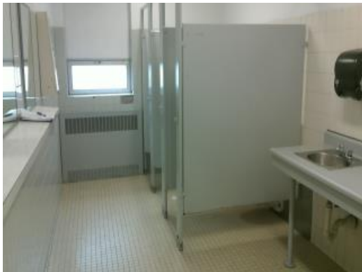
Restroom Fixtures And Finishes
