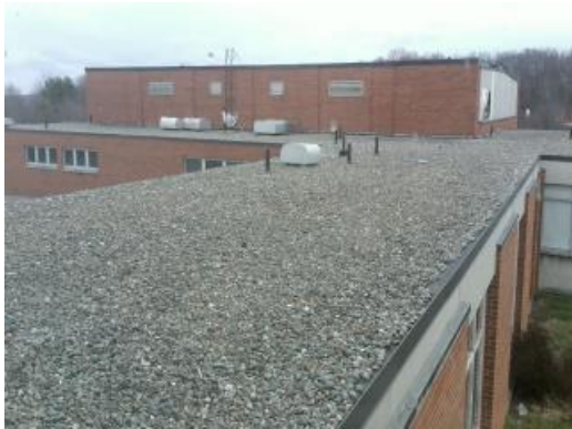
Ballasted Roof
