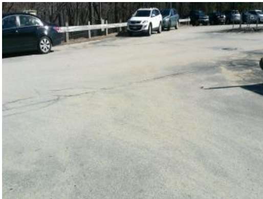
Weathered Asphalt
