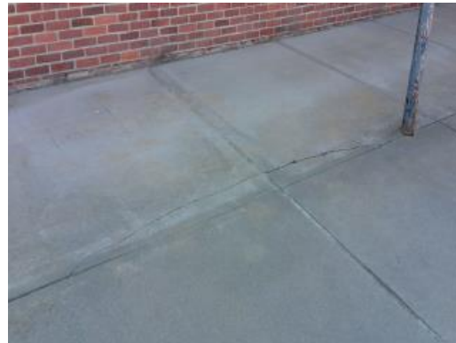
Sidewalk At North Entrance
