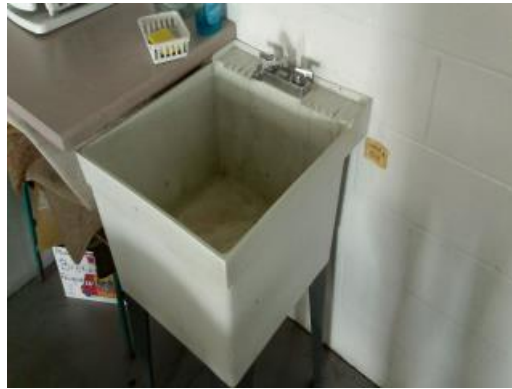
Stained Mop Sink
