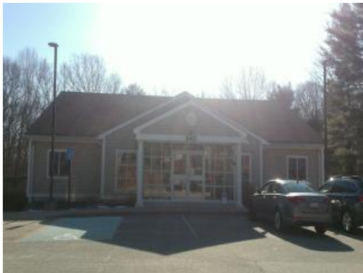
Building 02 - Front Elevation
