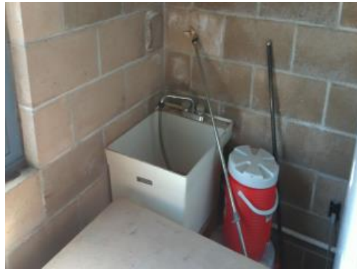
Building 04 - Mop Sink
