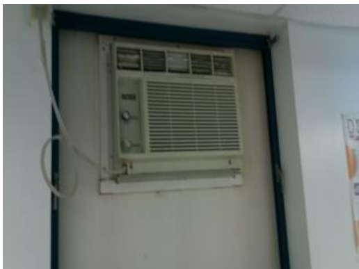
Main Building - Window Unit
