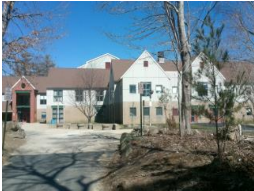
Main Building - East Elevation
