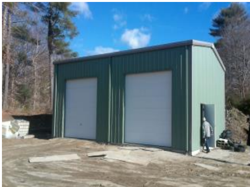
Building 03 - Exterior Elevation
