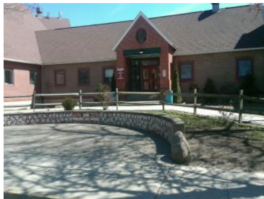
Main Building - West Elevation
