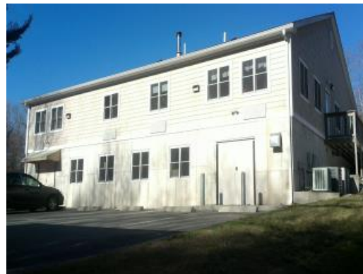
Building 02 - Rear Elevation
