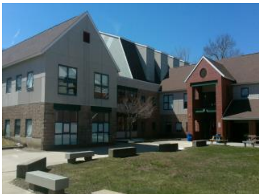
Main Building - Northeast Elevation
