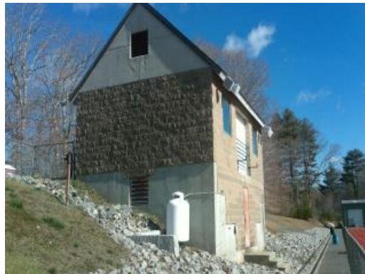
Building 04 - Pump House
