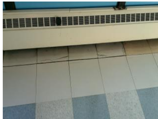
Separating VCT Flooring
