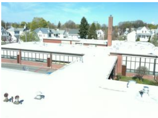
Roof General Condition
