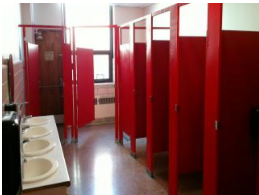
Restroom Fixtures And Finishes
