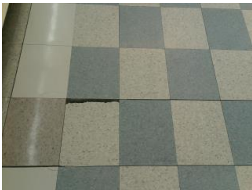
Separating VCT Flooring
