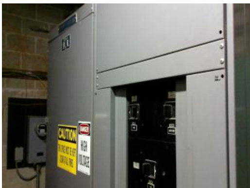
Main Switchgear
