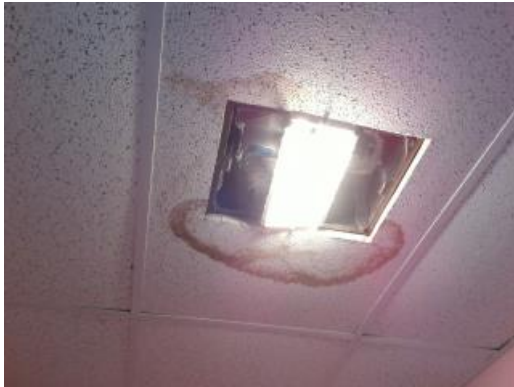
Girls Restroom Ceiling
