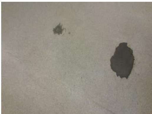
Epoxy Flooring at Kitchen
