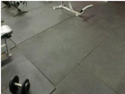
Worn Flooring at Weight Room
