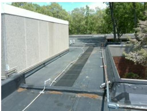
Typical Roof Condition
