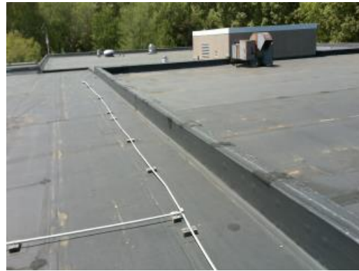
Typical Roof Condition
