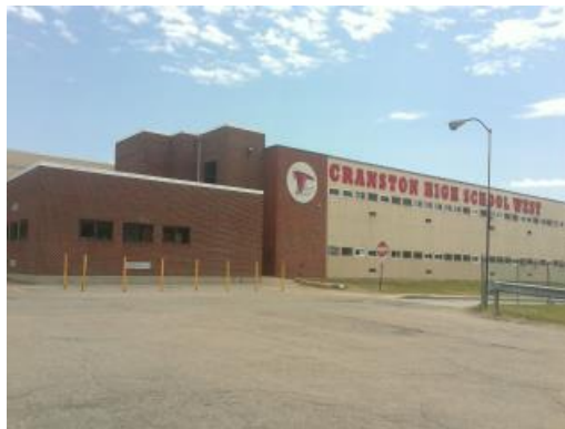
West Building Exterior
