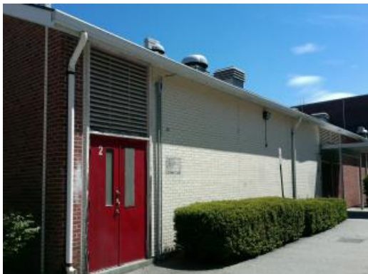
Auditorium Exterior Doors
