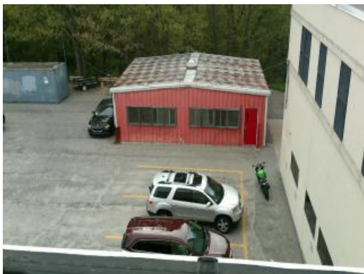
Metal Classroom Building
