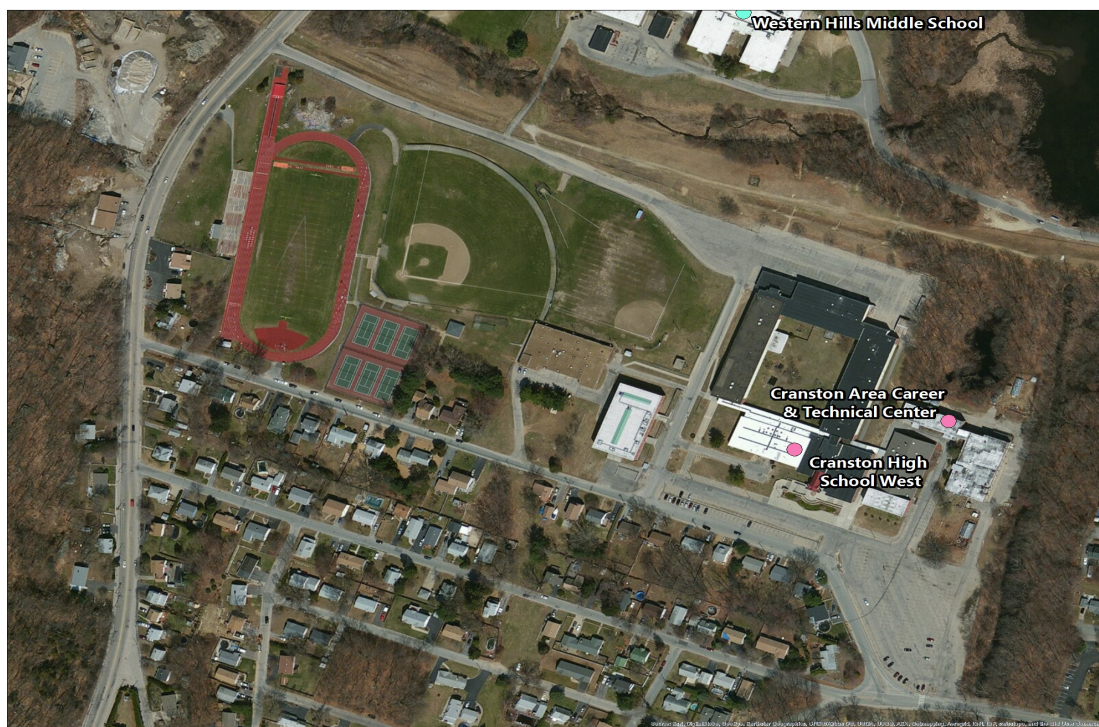
Figure 1: Aerial view of Cranston High School West
