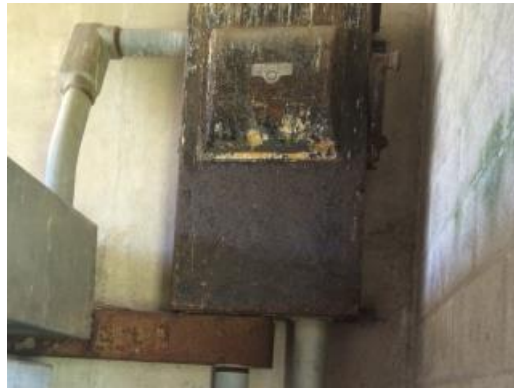
Corroded Disconnect
