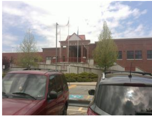
South Elevation Main Entrance
