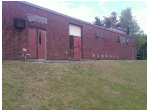
E Building Exterior
