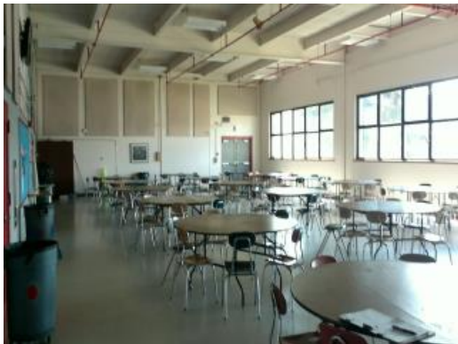
East Building Cafeteria
