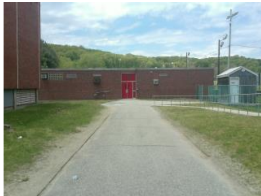
E Building Entrance
