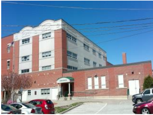
Side Of Building
