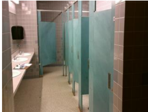
Toilet Room Gym Addition
