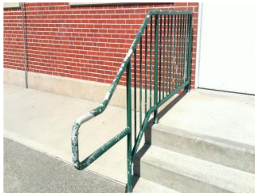
Peeling Handrail
