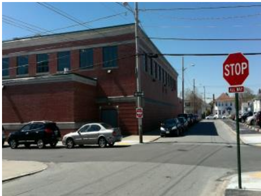
Side Of Building
