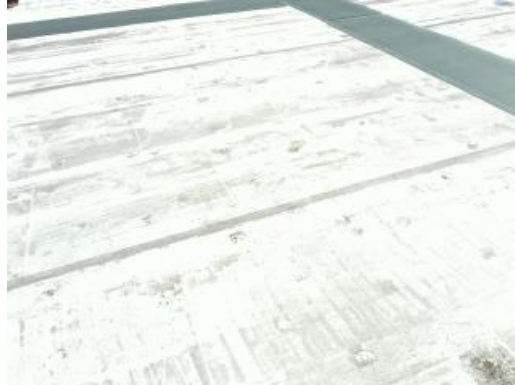
Weathered Roof Membrane
