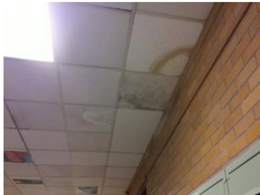
4th Floor Corridor Acoustical Ceiling Tiles
