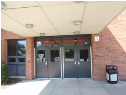
Exterior Entrance Doors
