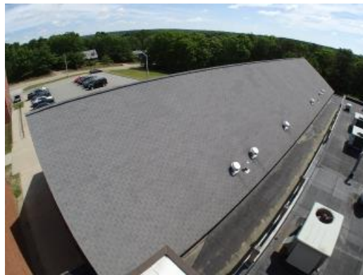
Composition Shingle Roof
