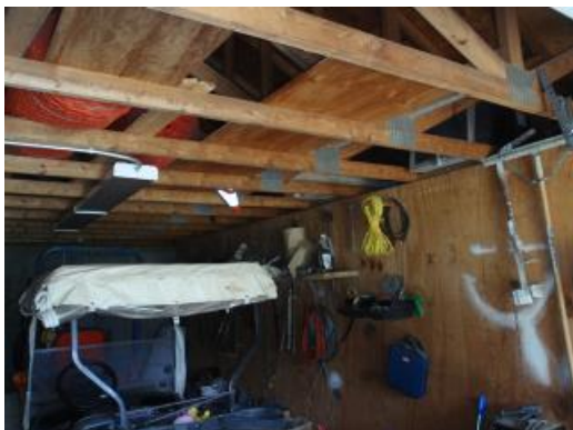
Storage Building Interior
