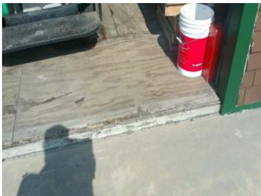
Building 5 Plywood Floor
