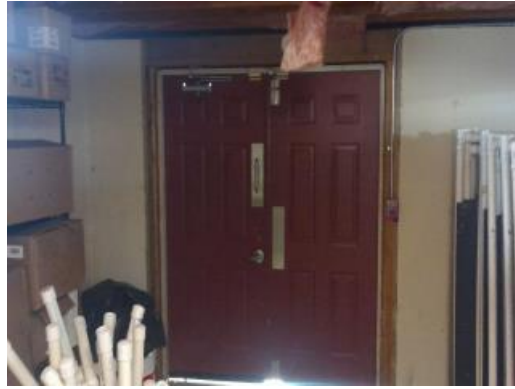
Admin Building Basement Exterior Doors
