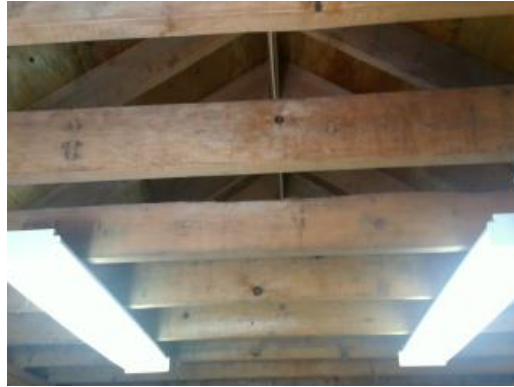
Building 6 Exposed Wood Ceiling
