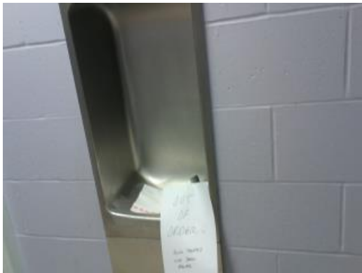
Broken Water Fountain
