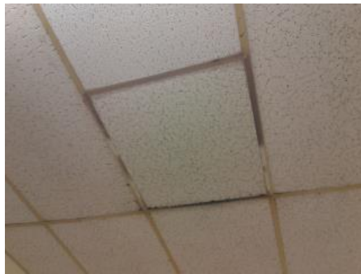
Stained Grid System
