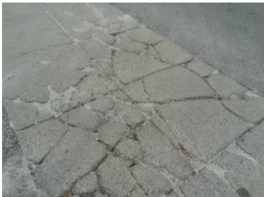
Cracked Sidewalk
