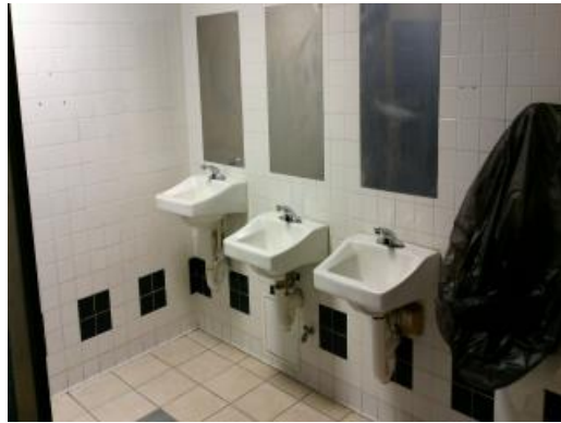
Typical Boys Restroom
