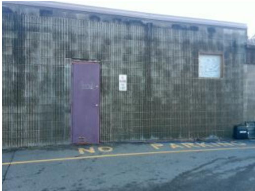
Maintenance Building Exterior
