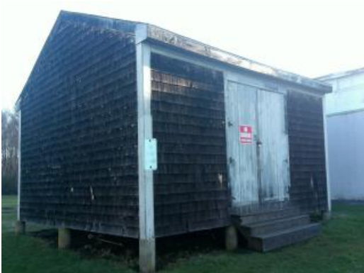
Weathered Wood Siding
