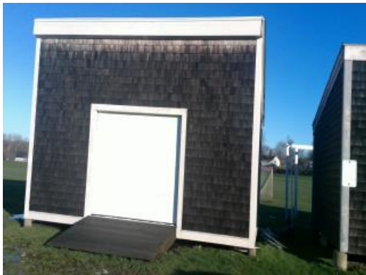
Storage Building 5 Exterior
