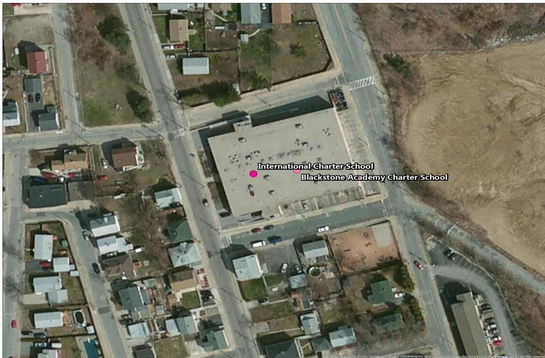
Figure 1: Aerial view of Blackstone Academy Charter School
