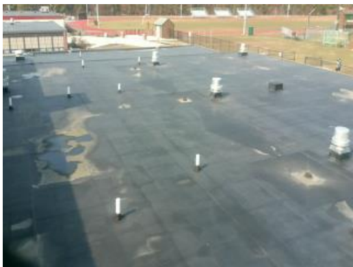
Main Building - Flat Roof
