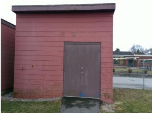
Building 04 - Secondary Field Storage
