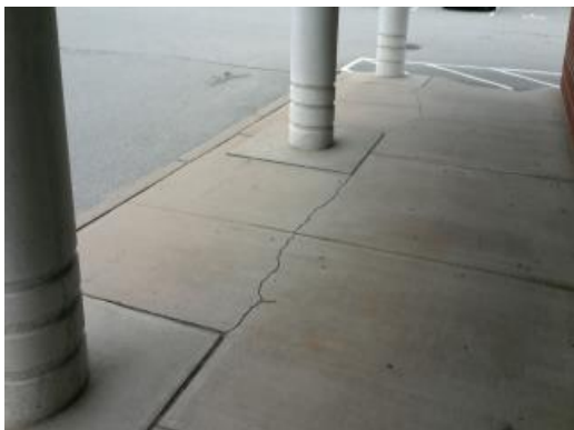
Main Building - Concrete Walk
