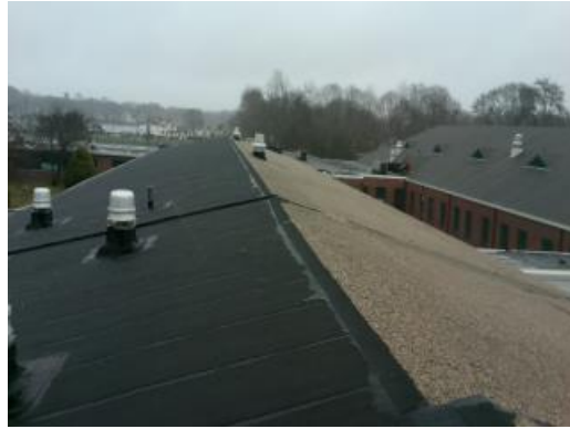
Main Building - Sloped Roof
