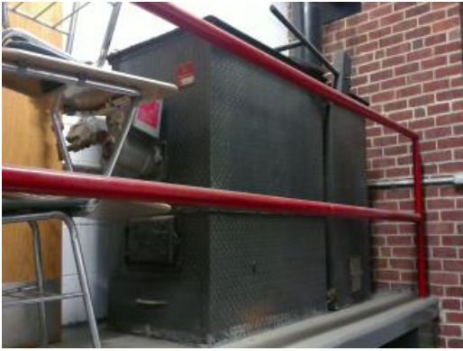
Main Building - Abandoned Incinerator
