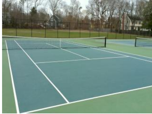
Site - Tennis Court
