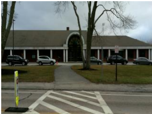
Main Building - Main Entry
