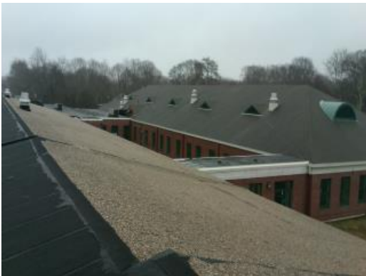
Main Building - Roof Exhausts
