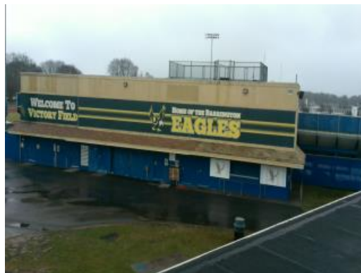
Building 02 - Stadium Elevation
