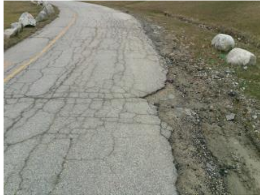
East Roadway Asphalt Paving
