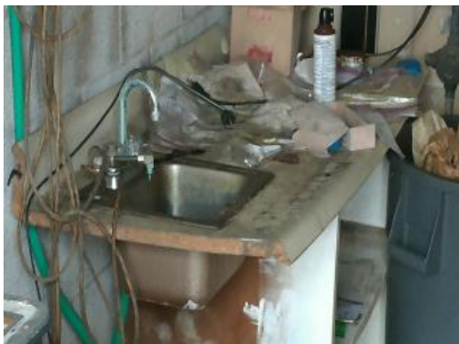
Septic House Lavatory
