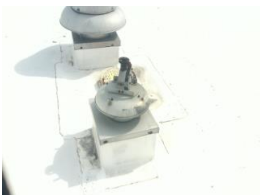
Damaged Small Exhaust Fan
