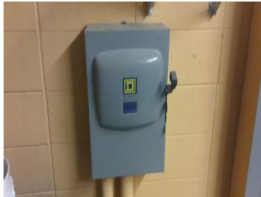
Transformer Disconnect
