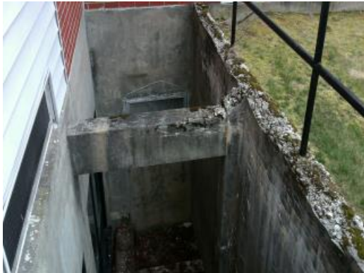
Courtyard Window Well
