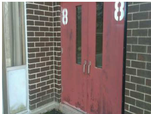
Original Exterior Doors
