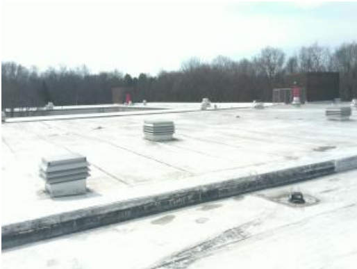
Roof General Condition
