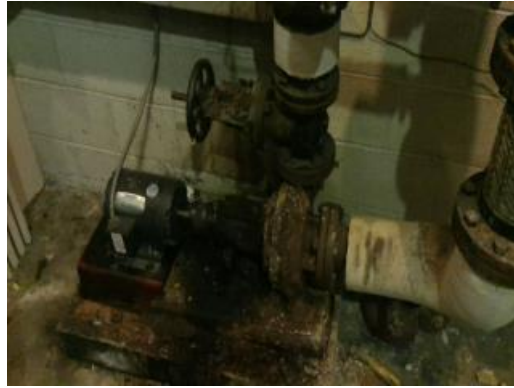
HVAC Circulating Pump
