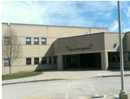
Drop Off Exterior
