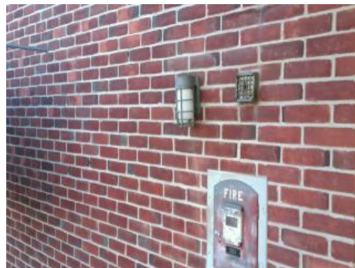
Aged Building Mounted Light
