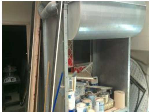
Lab Exhaust Hood
