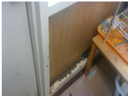
Rusted Window Frame
