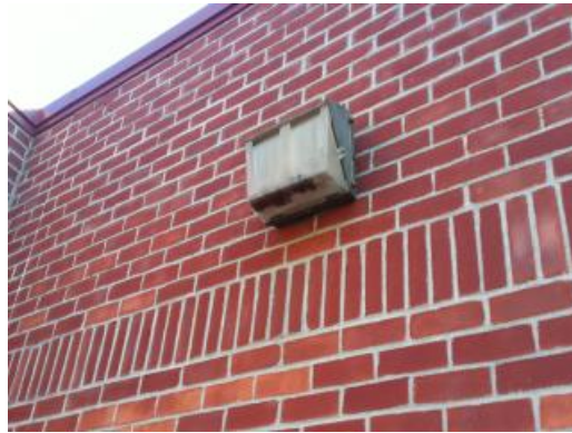
Aged Building Mounted Light
