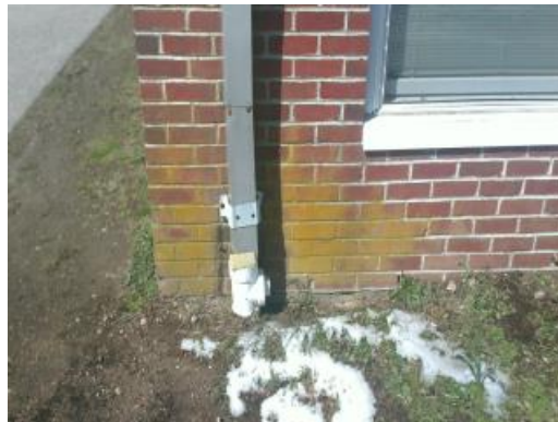
Leaking Downspout
