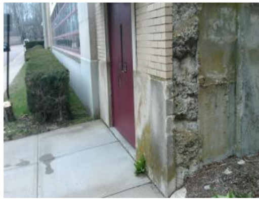
Concrete Wall Corner
