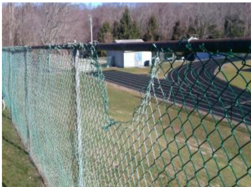
Damaged Chain Link Fence
