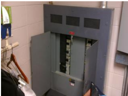
1,200 Amp Switchgear
