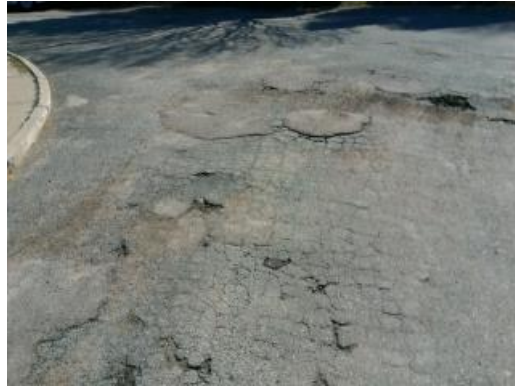
Alligatored Asphalt Paving
