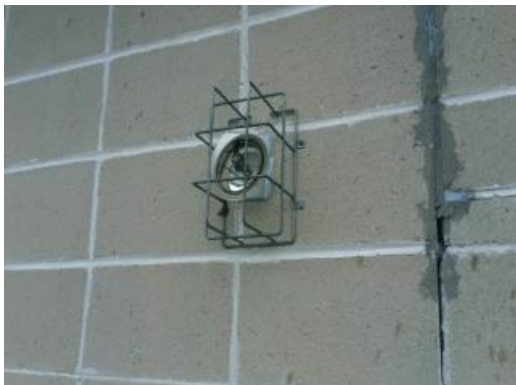
Low Efficiency Building Mounted Light
