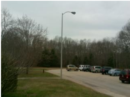
Parking Lot Lighting
