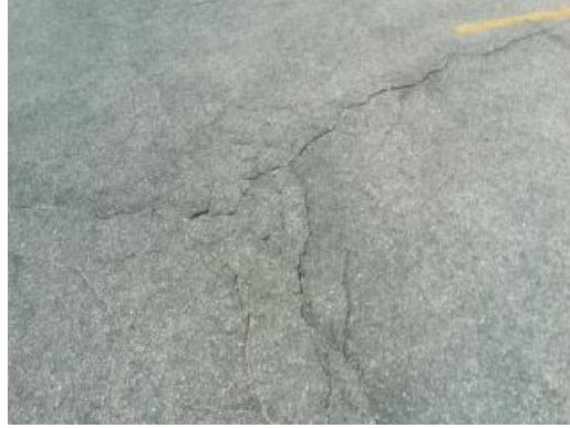
Splitting Asphalt Pavement
