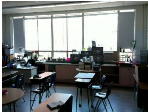
Single Pane Classroom Windows
