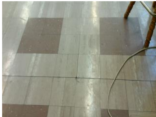
Separating VCT Flooring
