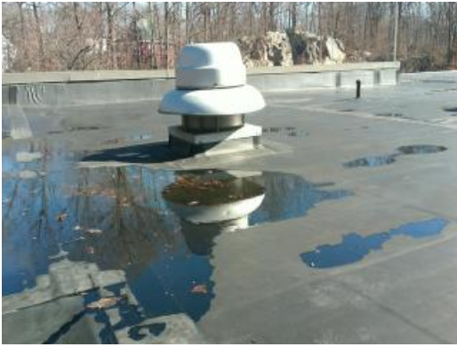
Large Exhaust Fan
