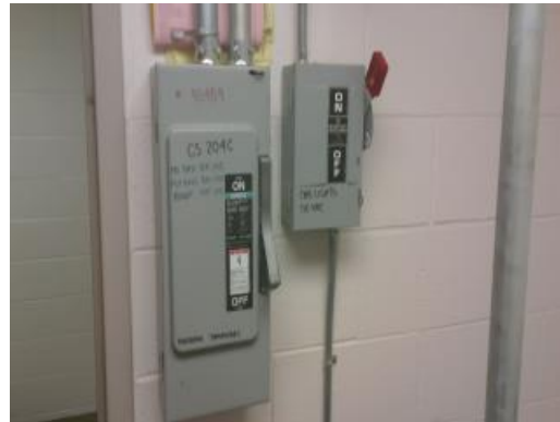
Elevator Disconnect
