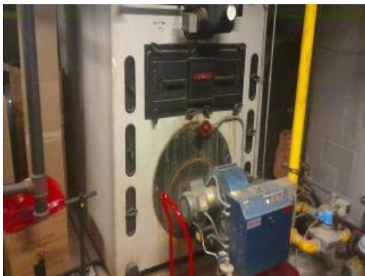
Corroded Boiler
