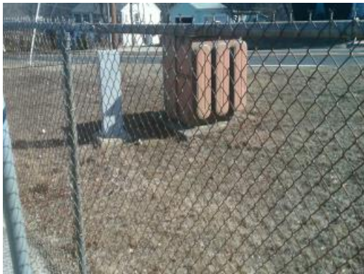
Chain Link Fencing
