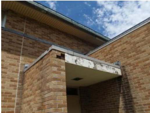
Damaged Brick
