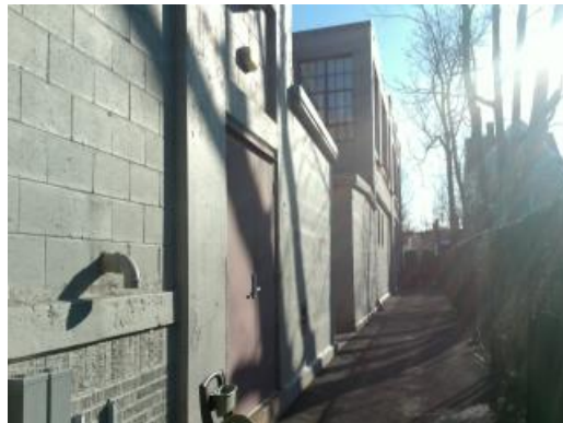
Rear of Building
