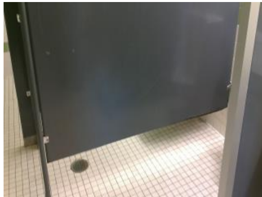
Typical Restroom Stall
