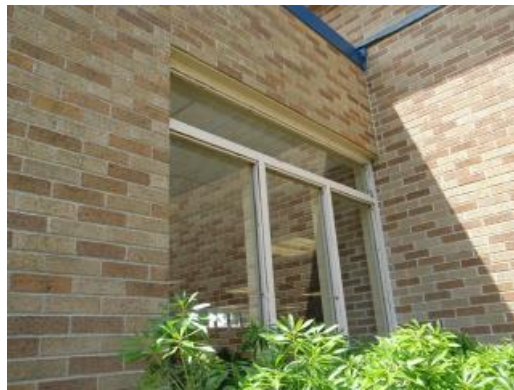
Aged Steel Windows
