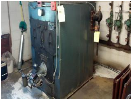
Leaking Boiler
