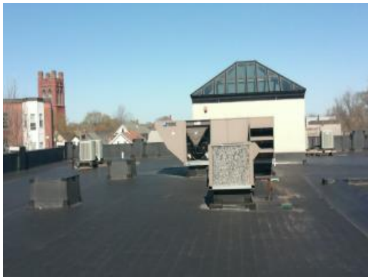
Typical Roof Condition
