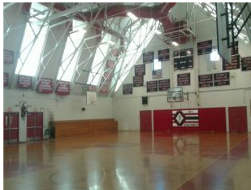
Main Building - Gymnasium
