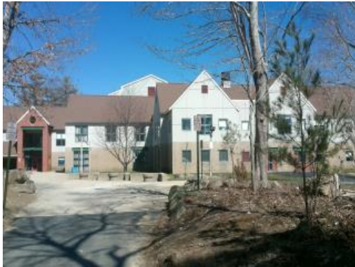
Main Building - East Elevation
