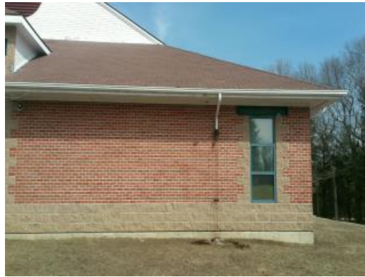
Missing Downspouts
