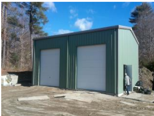
Building 03 - Exterior Elevation
