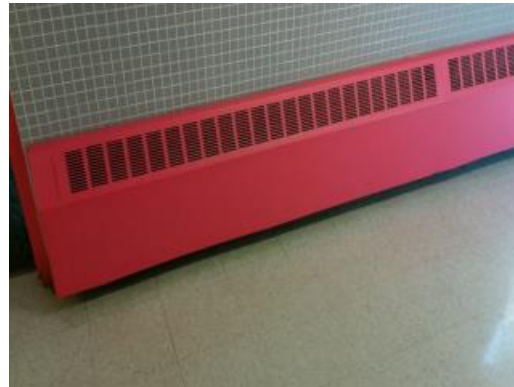
Radiant Wall Heater
