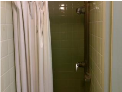
Original Shower Fixture
