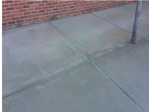
Sidewalk At North Entrance
