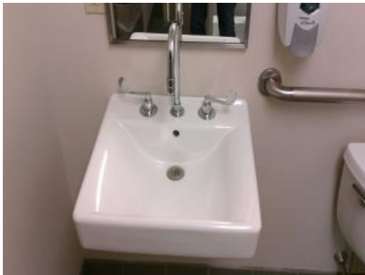
Building 02 - Typical Restroom Finish
