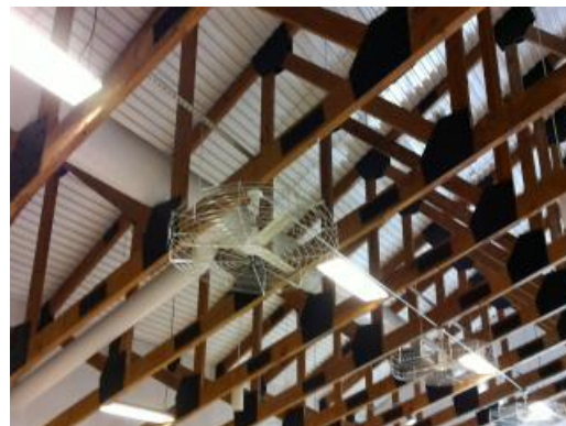
Cafeteria Exposed Ceiling
