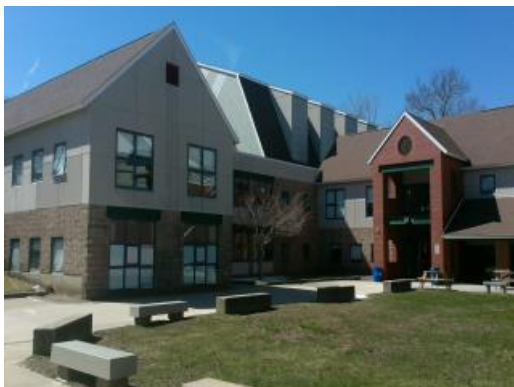
Main Building - Northeast Elevation
