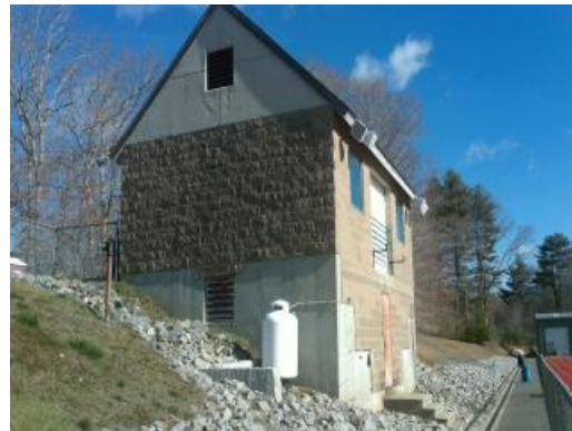
Building 04 - Pump House
