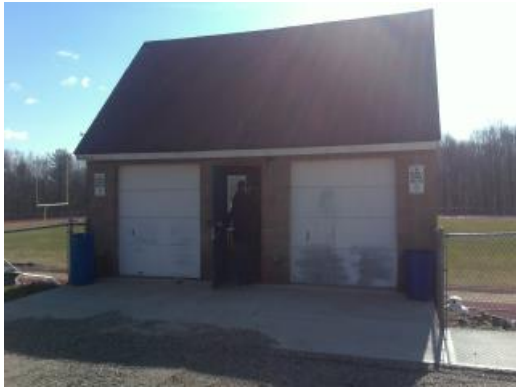
Building 04 - Concession Stand
