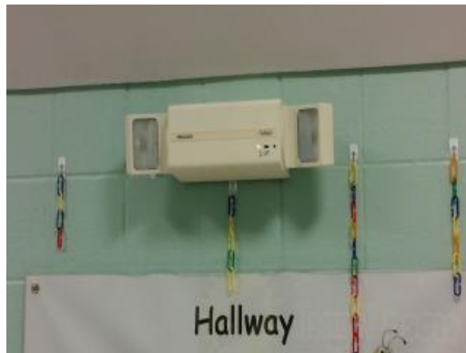
Battery Operated Emergency Light
