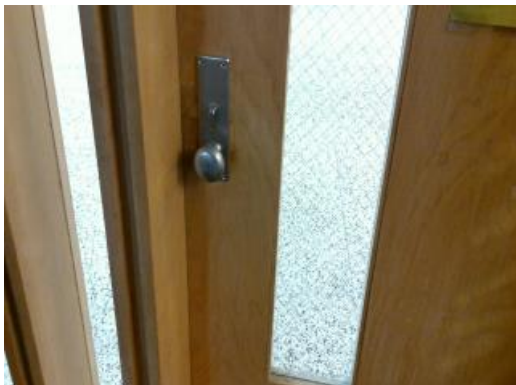
Typical Interior Door And Hardware
