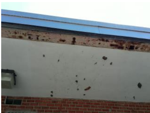
West Entry Soffit
