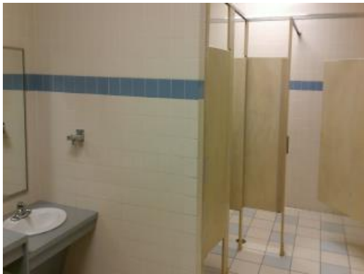
Restroom Fixtures And Finishes
