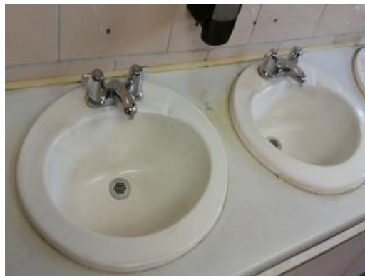
Typical Restroom Lavatories
