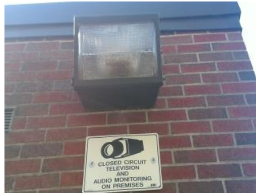
Mounted Building Light
