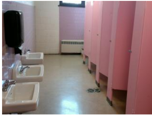
Restroom Fixtures And Finishse
