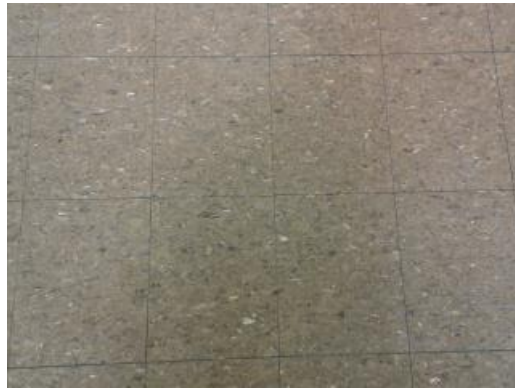
9x9 Tile In Gym/Cafeteria
