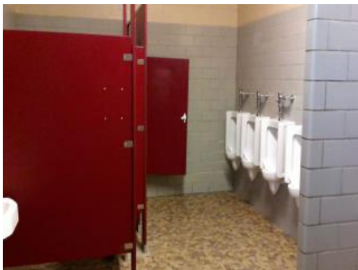
Typical Restroom Fixtures And Finishes
