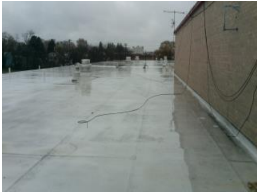
General Roof Condition
