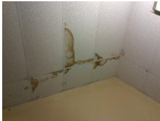
Stained Ceiling Tiles
