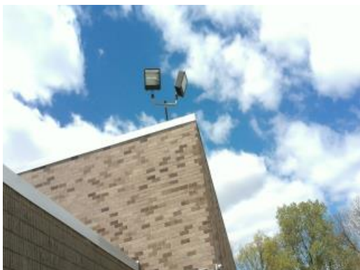
Aged Building Mounted Lights
