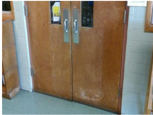
Typical Interior Wood Door.
