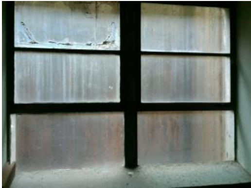
Original Basement Windows
