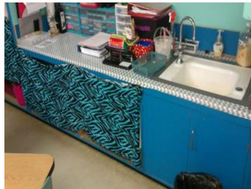
Aged Cabinetry Missing Doors
