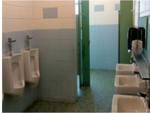
Restroom Fixtures And Finishes
