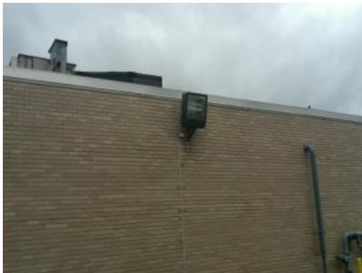
Building Mounted Light
