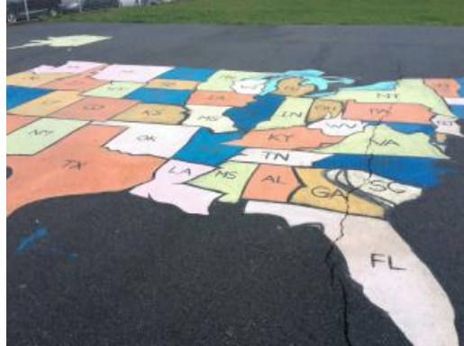
Cracked Play Area
