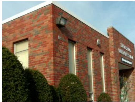
Building Mounted Lights
