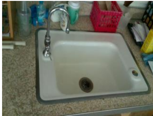
Typical Classroom Lavatory
