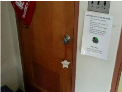
Typical Wood Door And Hardware
