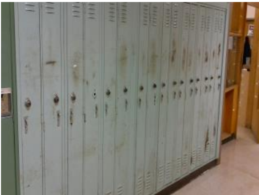
Typical Damaged Lockers
