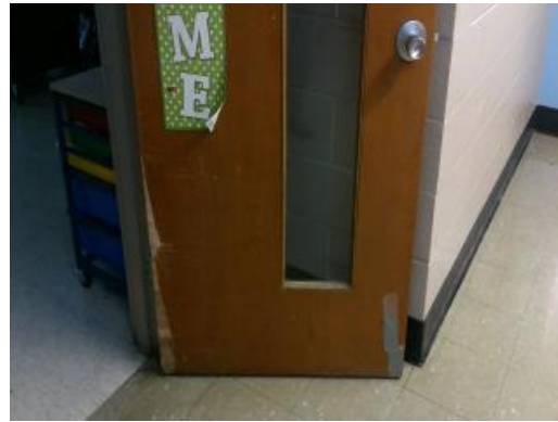
Worn Original Wood Door
