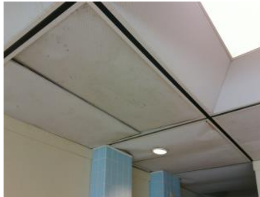
Metal Ceiling Panel
