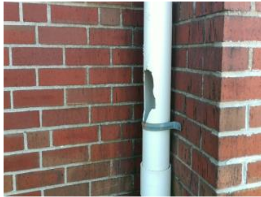
PVC Downspout On Southwest Corner
