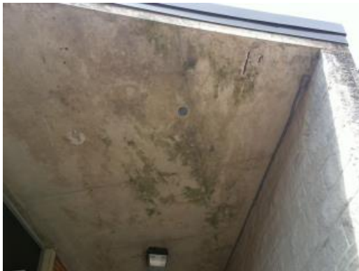
Stained Concrete Exterior
