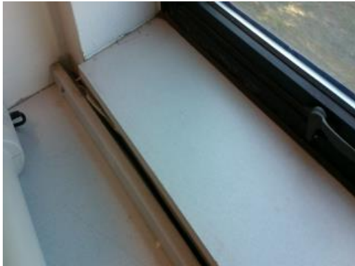
Delaminating Laminate
