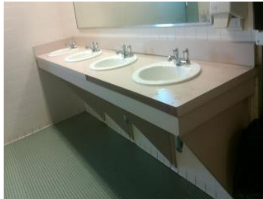
Delaminating Laminate
