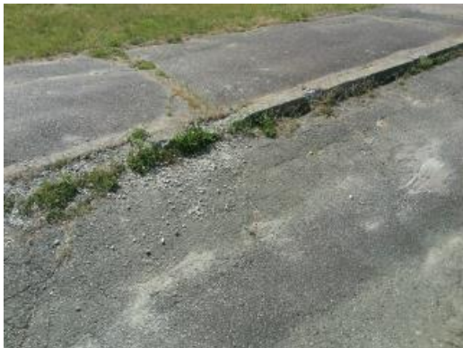
Deteriorated Curbs
