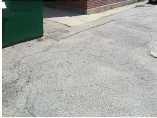
Weathered Asphalt
