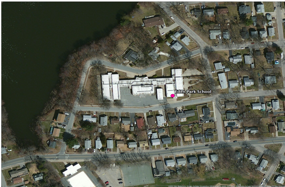
Figure 1: Aerial view of Eden Park School
