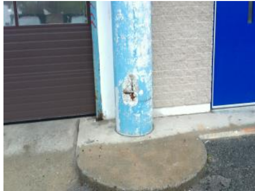
Damaged Column
