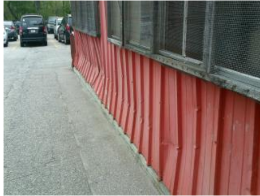
Damaged Facade
