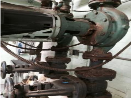
Corroded Pumps
