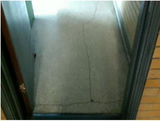
Cracking Terrazzo
