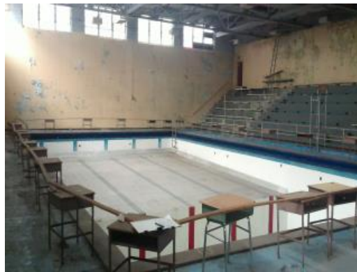
Abandoned Pool Area
