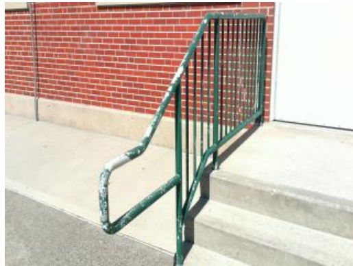
Peeling Handrail
