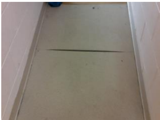
Lifting Rubber Floor
