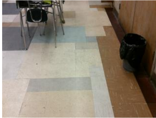
Vinyl Flooring In Classrooms
