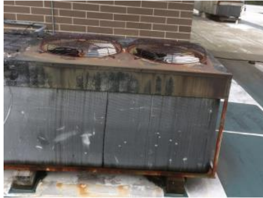
Weathered And Rusted Rooftop Unit
