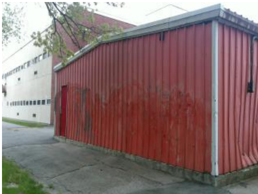
Damaged Facade
