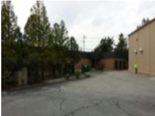
Main Building North Elevation
