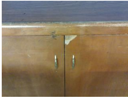
Typical Aged And Chipped Cabinetry
