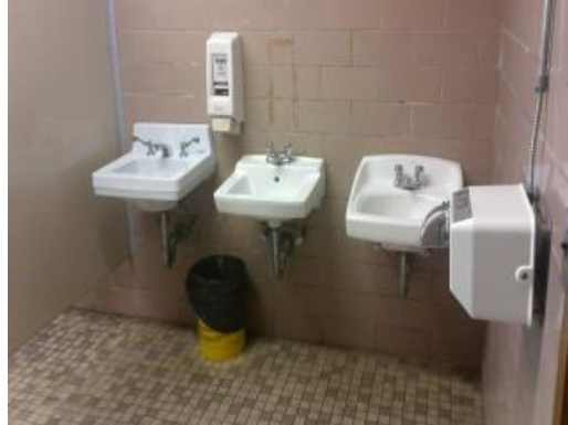
Restroom Finishes And Fixtures
