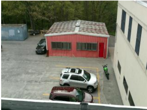
Metal Classroom Building
