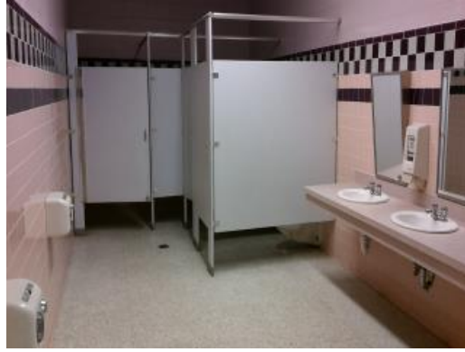
Restroom Fixtures And Finishes
