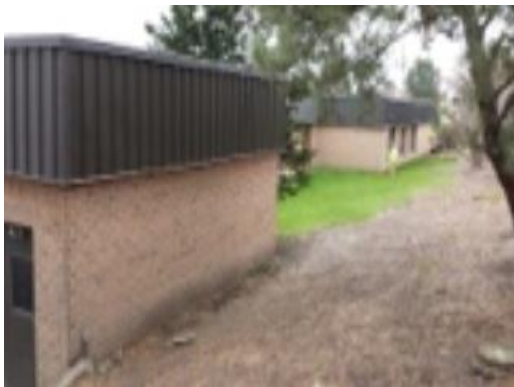
Main Building West Elevation
