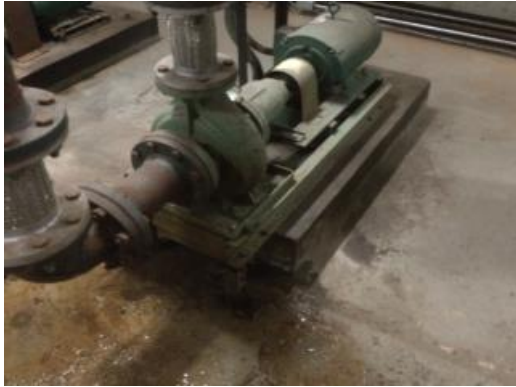
Leaking Pump
