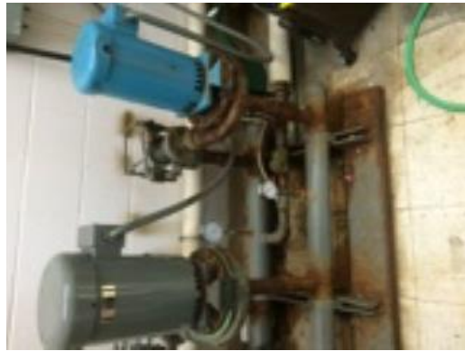
Leaking Pumps
