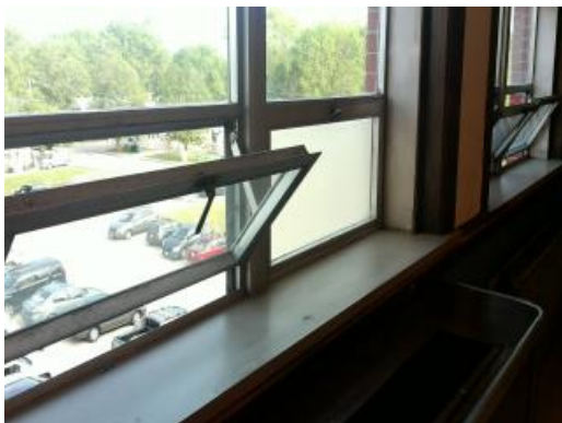
Typical Single Pane Windows
