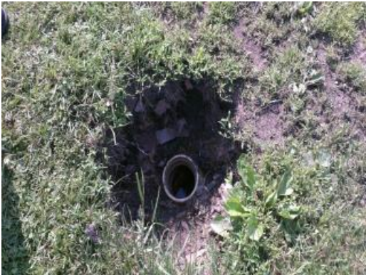
12" Deep Hole With Exposed Pipe
