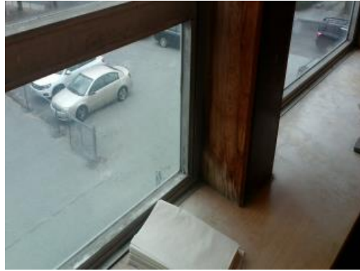
Typical Single-Pane Windows
