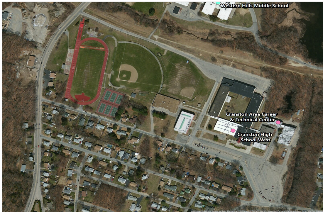
Figure 1: Aerial view of Cranston Area Career & Technical Center
