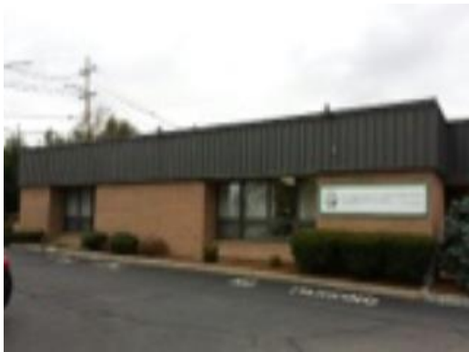
Main Building South Elevation
