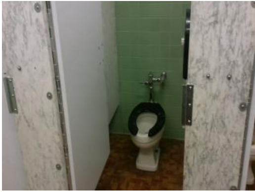
Typical Restroom Stall
