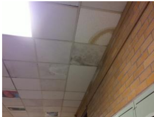
4th Floor Corridor Acoustical Ceiling Tiles
