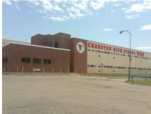
West Building Exterior
