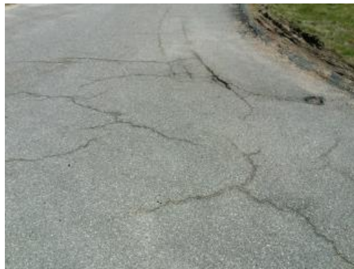
Cracked Asphalt
