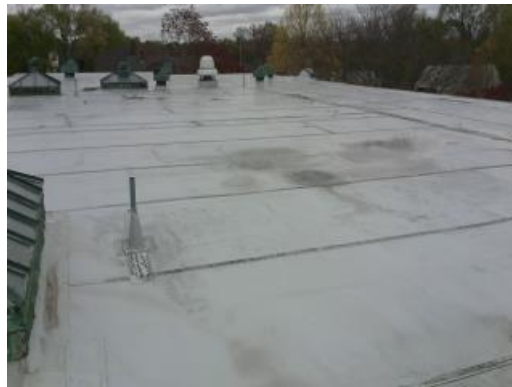
Single Ply Roofing
