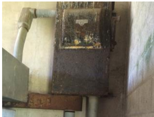
Corroded Disconnect
