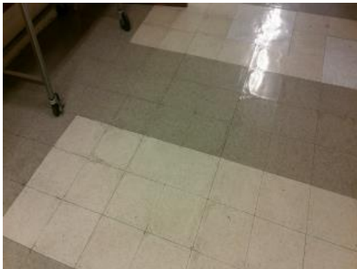
Worn VCT Bubbled At Seams
