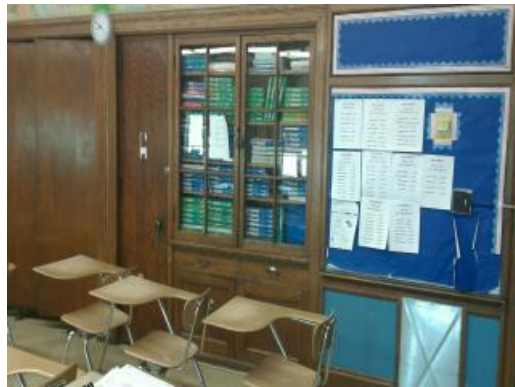
Typical Built-In Casework
