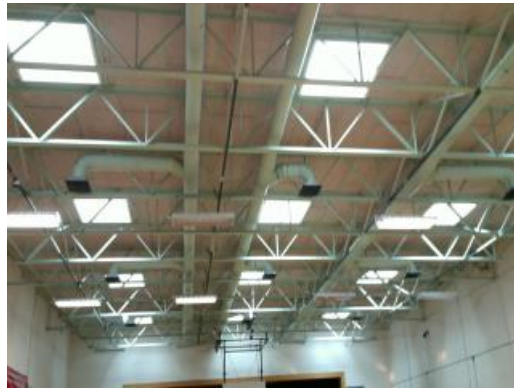
Exposed Gym Ceiling
