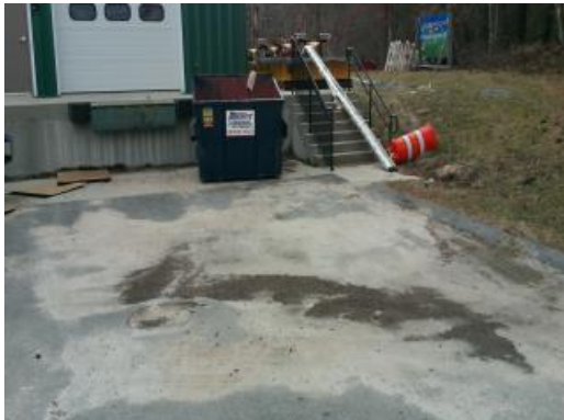
Building 2 Loading Dock
