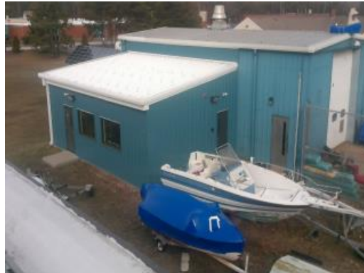
Marine Building Exterior
