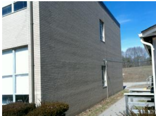
Exterior Brick Wall
