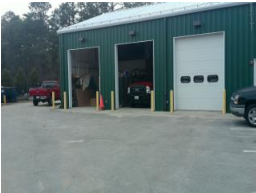
Building 2 Garage Bays
