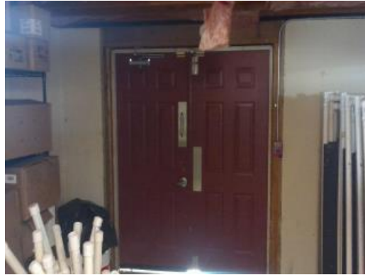
Admin Building Basement Exterior Doors
