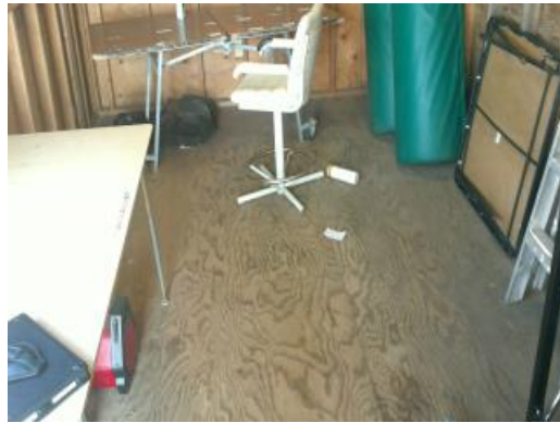
Building 6 Wood Floor
