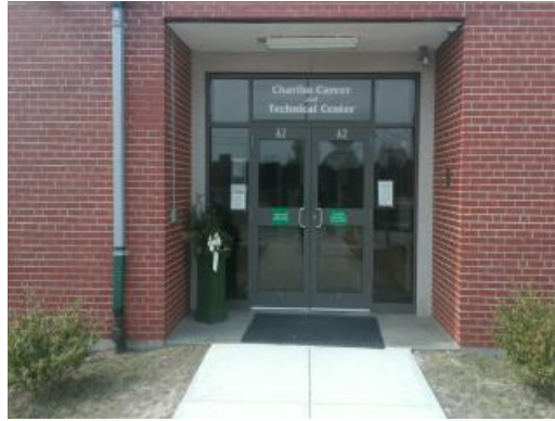
Entrance Way Signage
