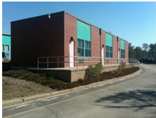
Addition Classrooms Exterior
