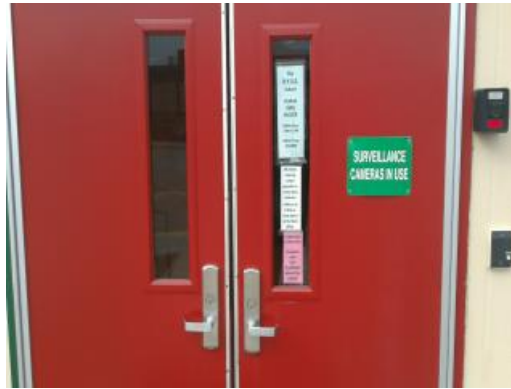
Front Entrance Doors
