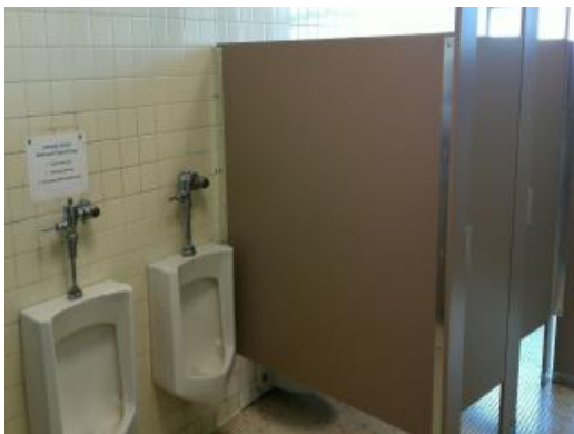
Restroom Fixtures And Finishes
