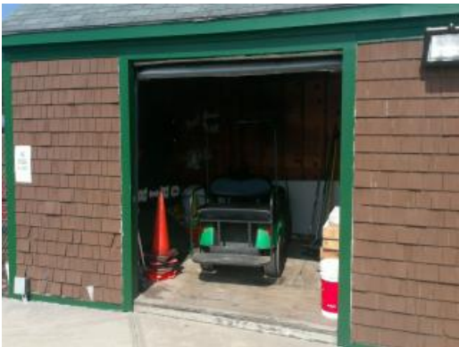
Building 5 Overhead Door
