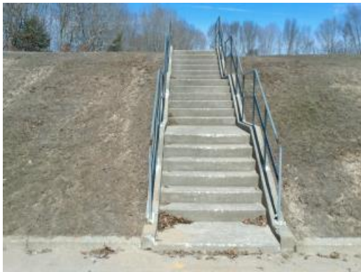
Concrete Stairs To Field
