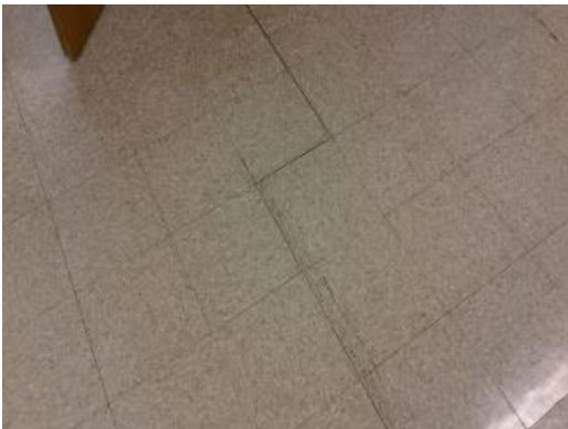
Separating VCT Flooring
