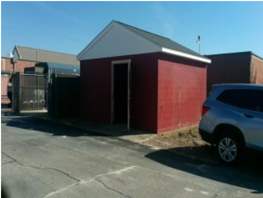
Storage Building Exterior
