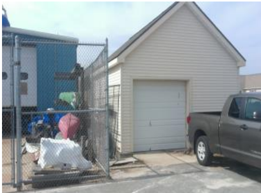
Storage Building Exterior
