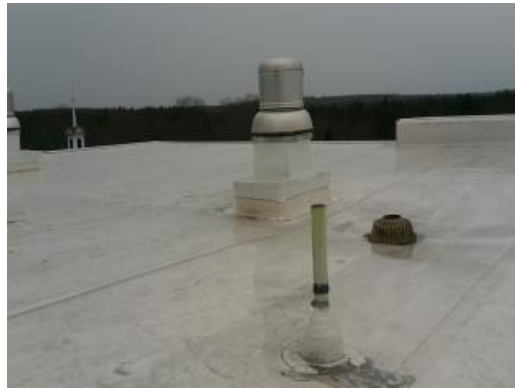
General Roof Condition
