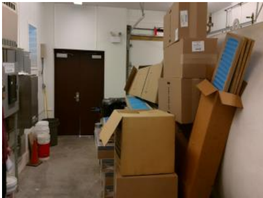
Water Tank Room
