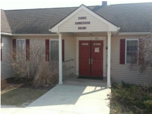
Admin Building Main Entrance
