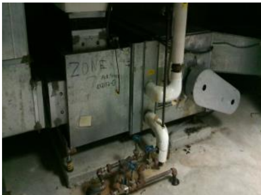
Heating and Ventilating Unit
