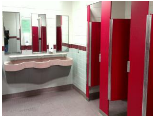
Restroom Fixtures And Finishes
