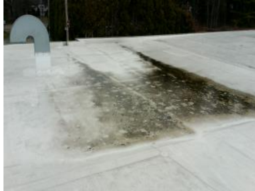
Damaged EPDM
