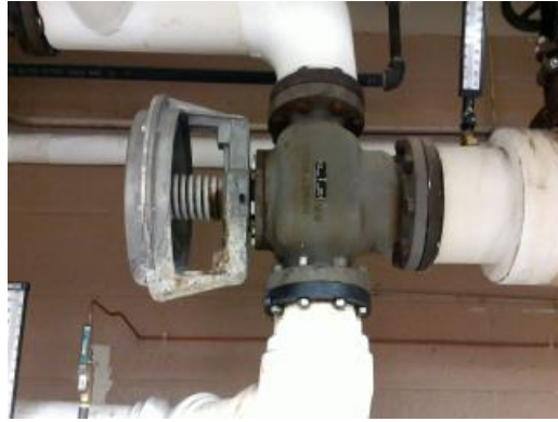
Heating Hot Water Control Valve
