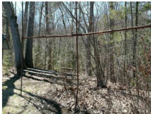
Rusted and Damaged Fence
